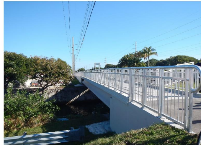
Monroe County - Marvin Adams Pedestrian Bridge
