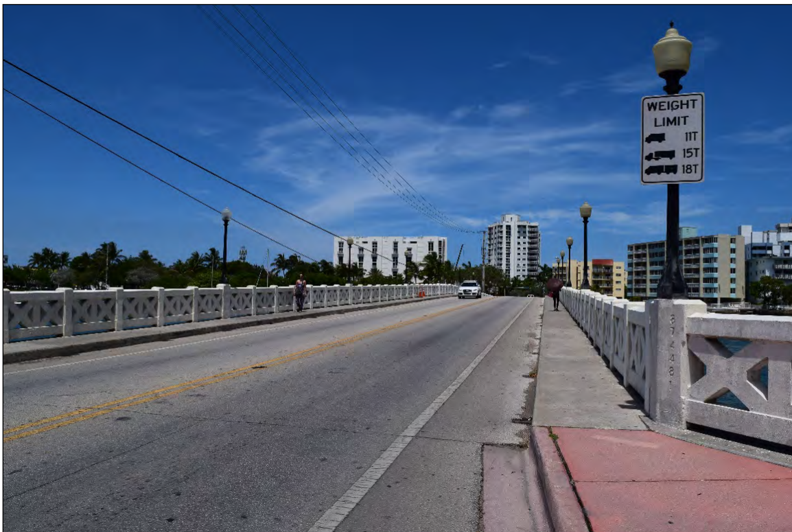
Figure 7: Existing Concrete Decking, Sidewalks, and Railings within the Archaeological APE at Venetian Causeway Bridge 12 (8DA14384), Facing East
