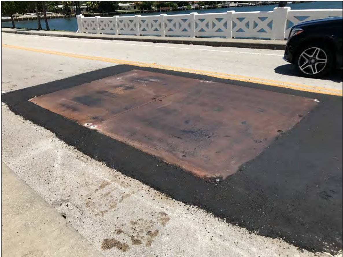
FIGURE 4: BRIDGE DECK FAILURE AND REPAIR
