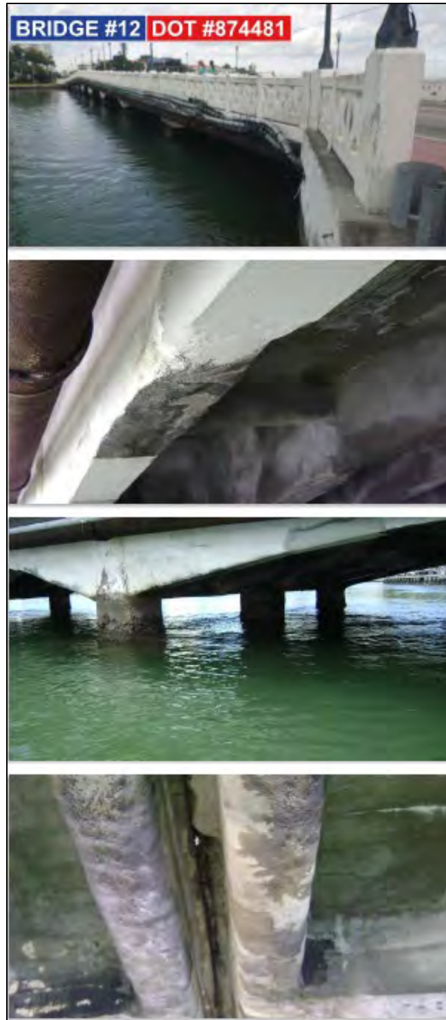
Figure 18: Bridge 12 Current Conditions
