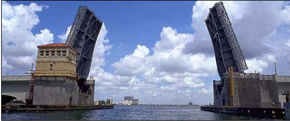
Figure 3: Bridge 1 Double-Leaf Bascule Span
