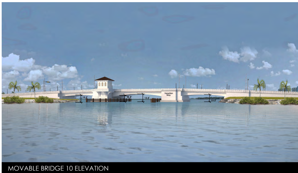
Figure 1-20 Replacement Alternative M4: Double Leaf Bascule Bridge
