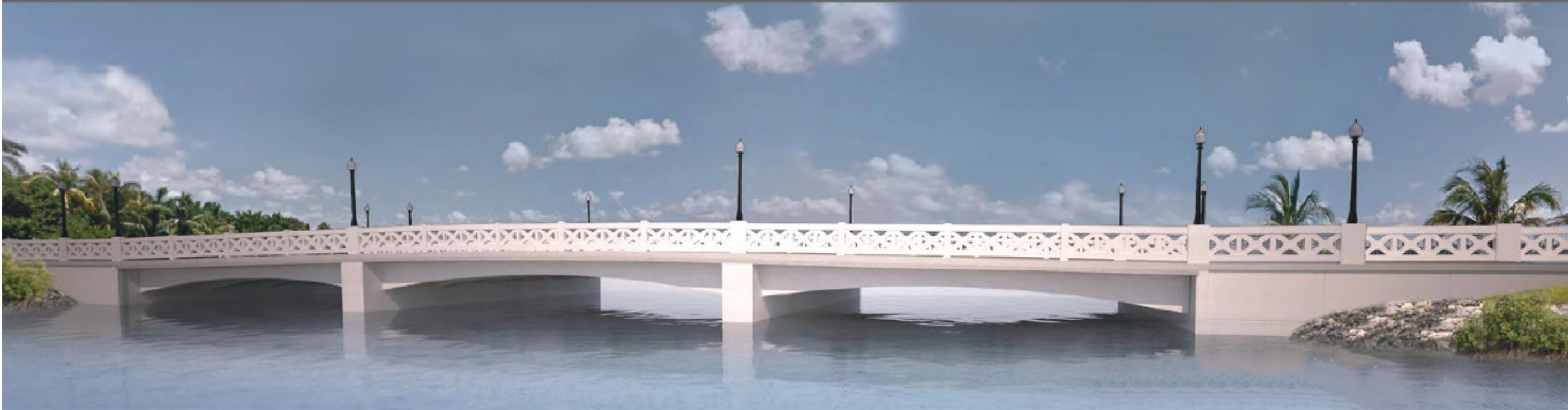
Fixed Bridge Alternative 7 — Arched Beams
