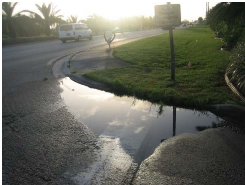
This picture depicts the existing pavement, drainage and pavement markings along the study corridor. As can be seen in the picture taken along SW 8 th Street, east of SW 87 th Avenue, the study area facility is in poor to fair conditions
