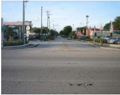
South view of the northbound approach of the intersection of SW 8 th Street and SW 86 th Avenue
