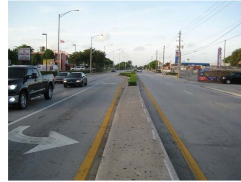
View of the median along SW 87 th Avenue south of SW 8 th Street. FPL overhead utilities are located on the eastern side of the road.
