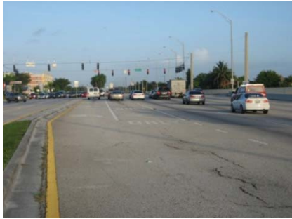
West view of the westbound approach of SW 87 th Avenue and SW 8 th Street
