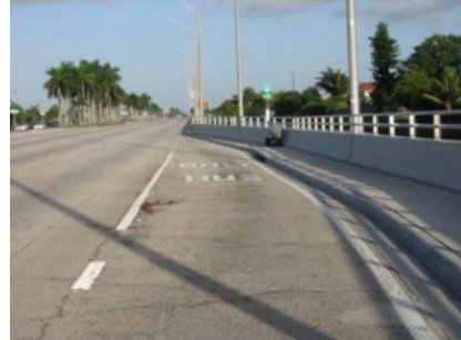
View of the bus bay located on the northwestern corner of the intersection of SW 87 th Avenue and SW 8 th Street
