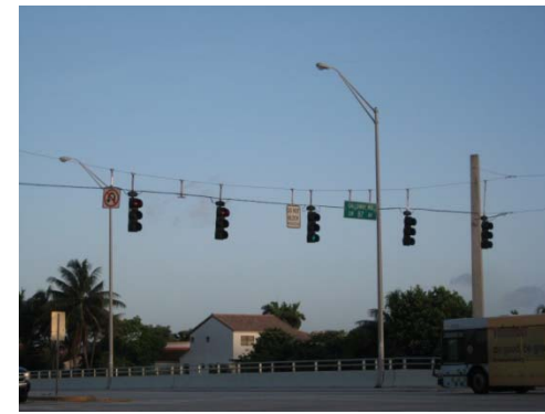
Southwesterly view of the signal of SW 8 th Street and SW 87 th Avenue. The signal is currently mounted on span wire.
