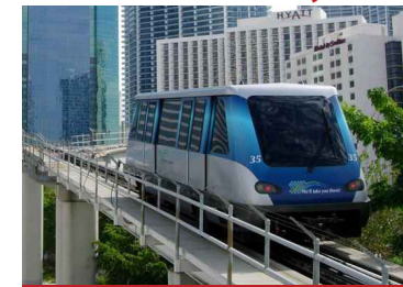
Metromover - Automated People Mover (APM)
