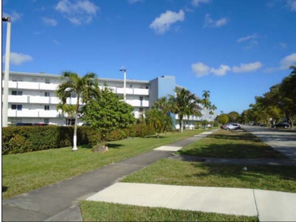
Figure 11 – 215: Rolling Green Condo H (1101 NE 191 st Street) (8DA21541), c. 1970, Considered National Register-Ineligible, facing East
