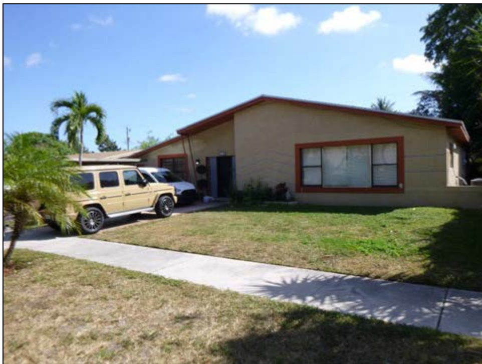
Figure 11 – 37: 370 East Drive (8DA14242), Determined National Register-Ineligible, facing Southeast
