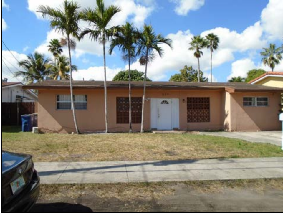
Figure 11 – 244: 520 SW 11 th Avenue (8BD8589), c. 1961, Considered National Register-Ineligible, facing West
