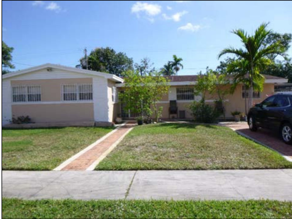
Figure 11 – 46: 470 East Drive (8DA14251), Determined National Register-Ineligible, facing Southeast
