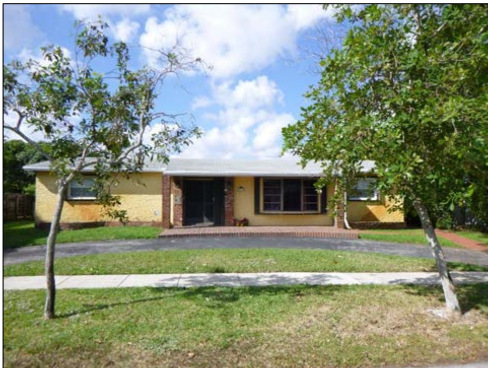
Figure 11 – 59: 18300 NE 7 th Court (8DA14268), Determined National Register-Ineligible, facing West
