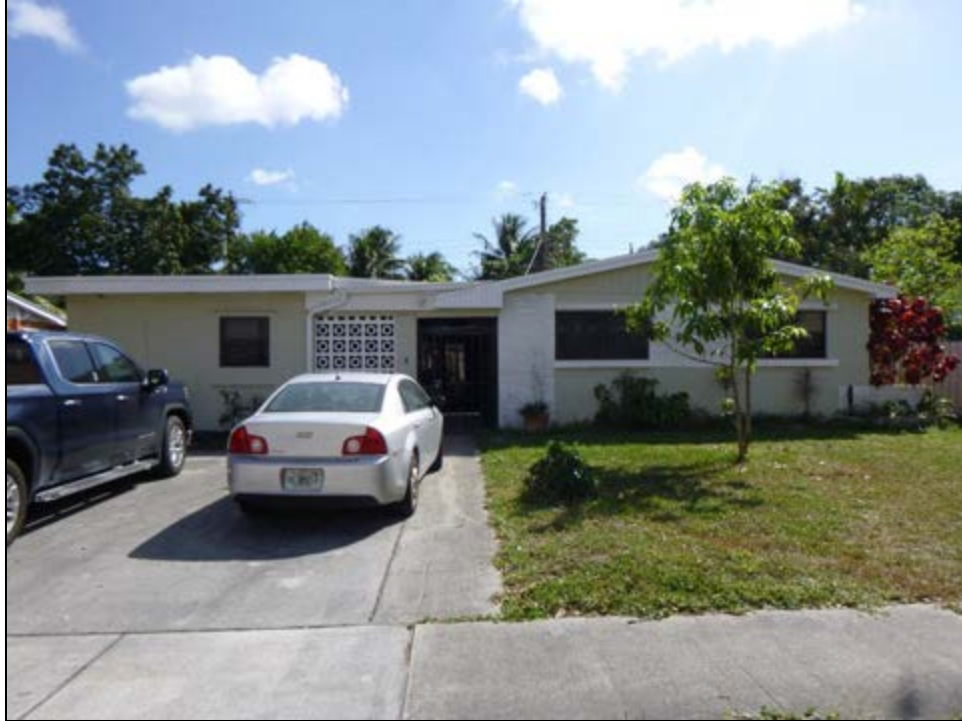
Figure 11 – 20: 180 East Drive (8DA14225), Determined National Register-Ineligible, facing Southeast
