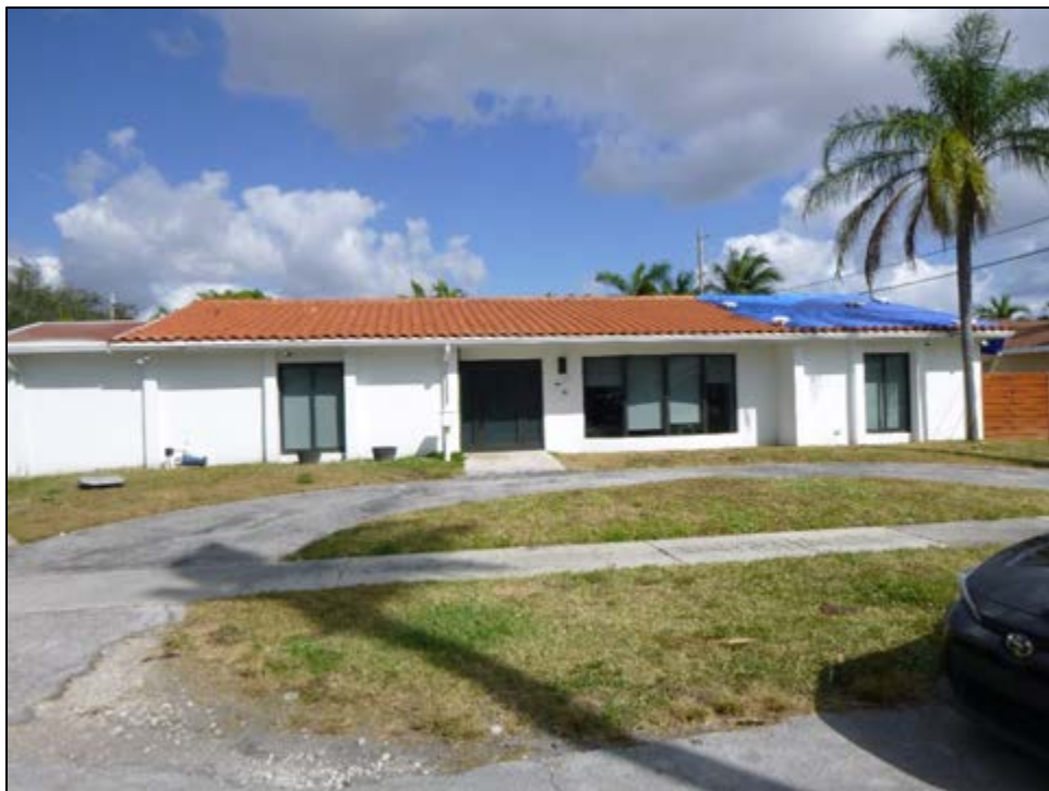
Figure 11 – 198: 1865 NE 208 th Terrace (8DA21503), c. 1973, Considered National Register-Ineligible, facing North
