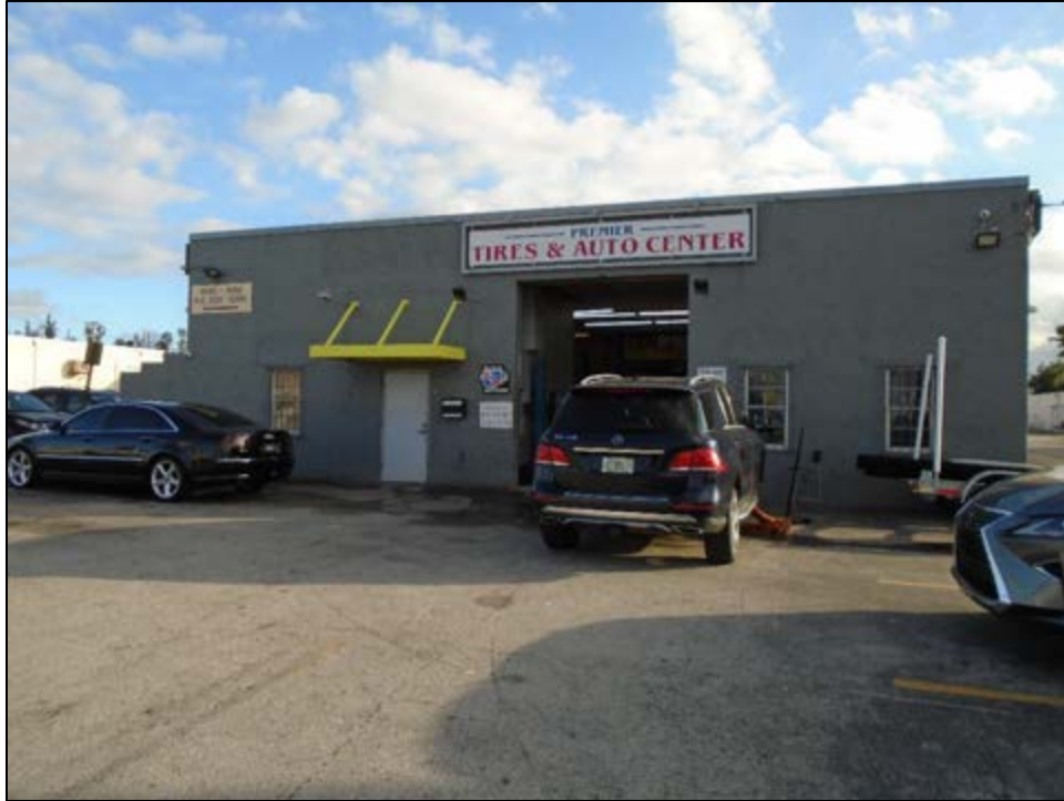
Figure 11 – 218: Ronson Industrial Park (8DA21543), c. 1973, Considered National Register-Ineligible, facing South
