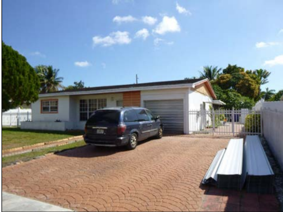
Figure 11 – 24: 230 East Drive (8DA14229), Determined National Register-Ineligible, facing Southeast
