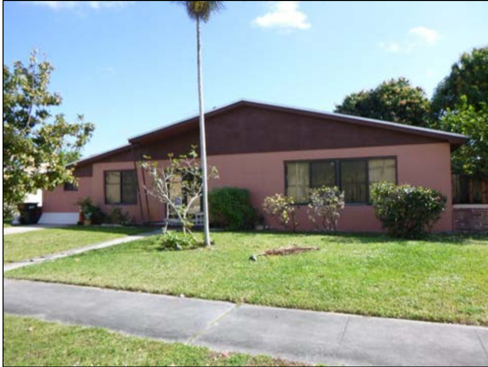
Figure 11 – 48: 490 East Drive (8DA14253), Determined National Register-Ineligible, facing Southeast
