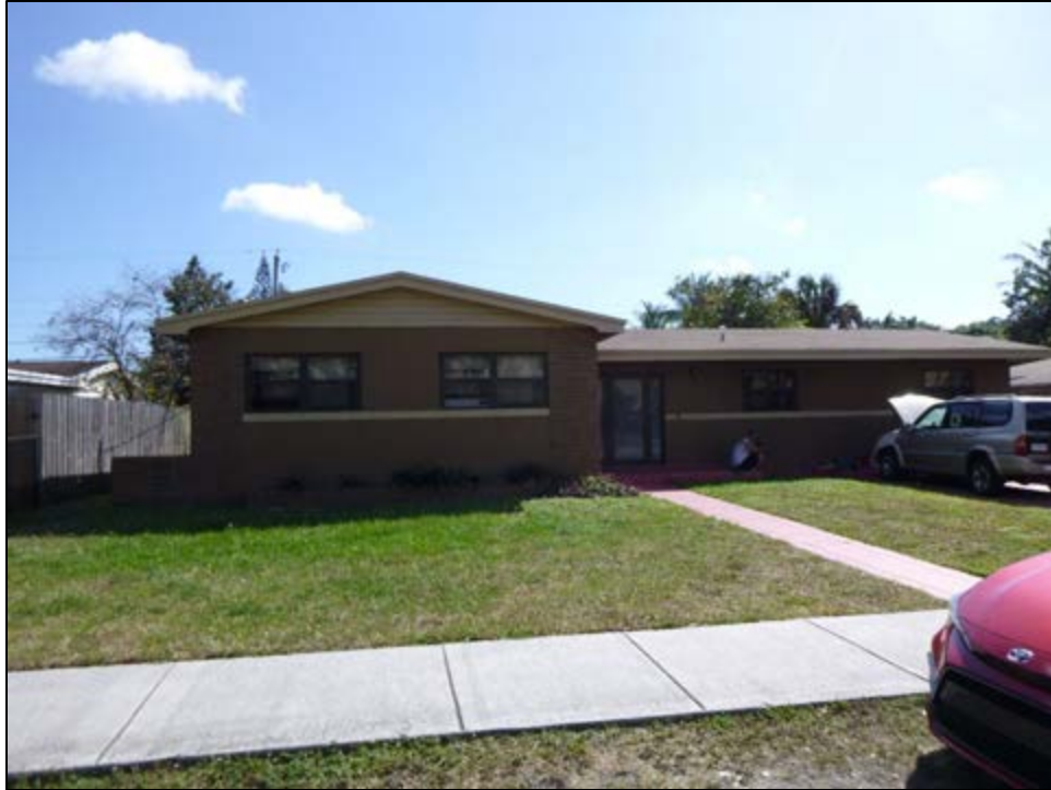
Figure 11 – 38: 380 East Drive (8DA14243), Determined National Register-Ineligible, facing Southeast
