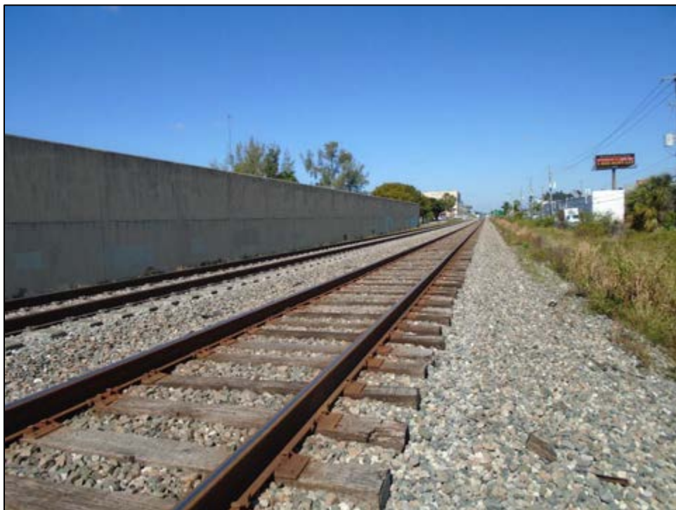
Figure 11 – 71: Seaboard Air Line (CSX) Railroad (8BD4649) Within the APE, Determined National Register-Eligible, facing North
