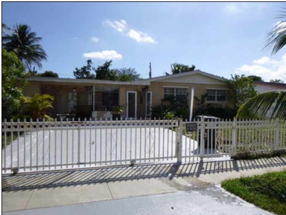
Figure 11 – 25: 240 East Drive (8DA14230), Determined National Register-Ineligible, facing Southeast
