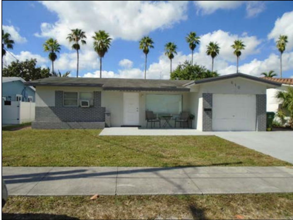
Figure 11 – 240: 610 SW 11 th Avenue (8BD8585), c. 1963, Considered National Register-Ineligible, facing West
