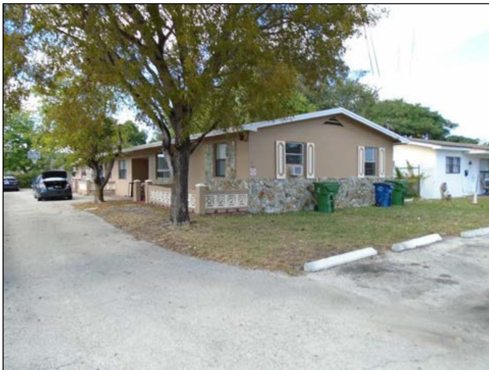
Figure 11 – 253: 340 SW 11 th Avenue (8BD8597), c. 1961, Considered National Register-Ineligible, facing Northwest
