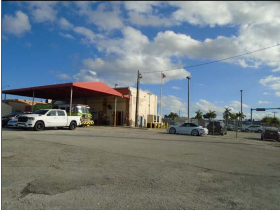
Figure 11 – 153: Miami Dade Fire Rescue Station #63 (1655 NE 205 th Street) (8DA21461), c. 1968, Considered National Register-Ineligible, facing Southeast
