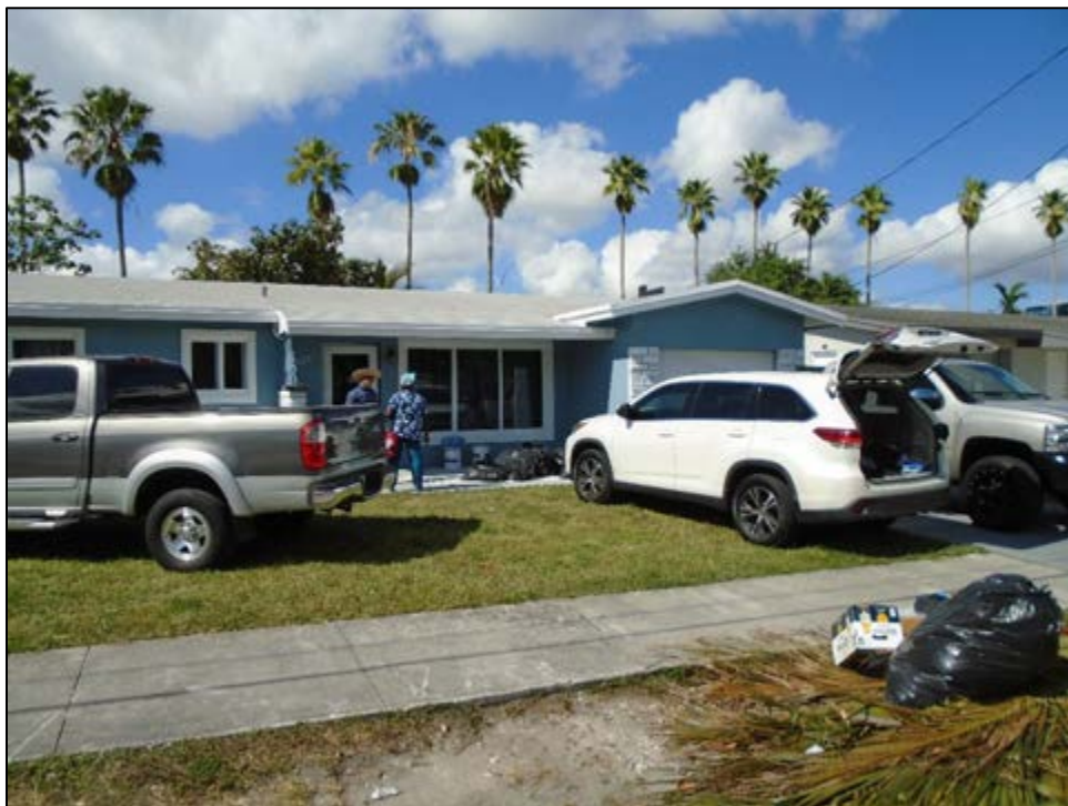
Figure 11 – 239: 620 SW 11 th Avenue (8BD8584), c. 1962, Considered National Register-Ineligible, facing West
