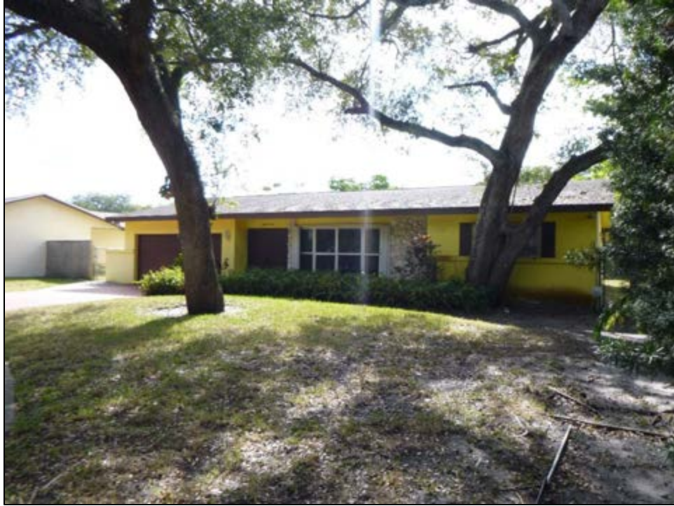
Figure 11 – 193: 1860 NE 206 th Terrace (8DA21498), c. 1975, Considered National Register-Ineligible, facing Southeast
