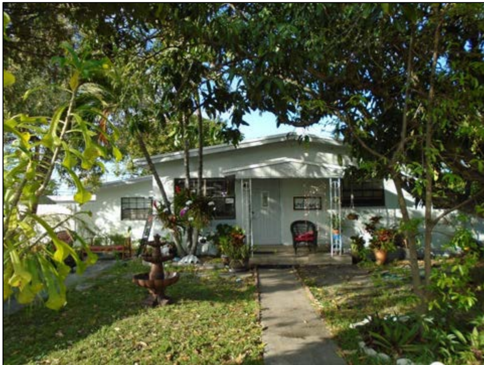
Figure 11 – 160: 1521 NE 205 th Terrace (8DA21467), c. 1956, Considered National Register-Ineligible, facing North
