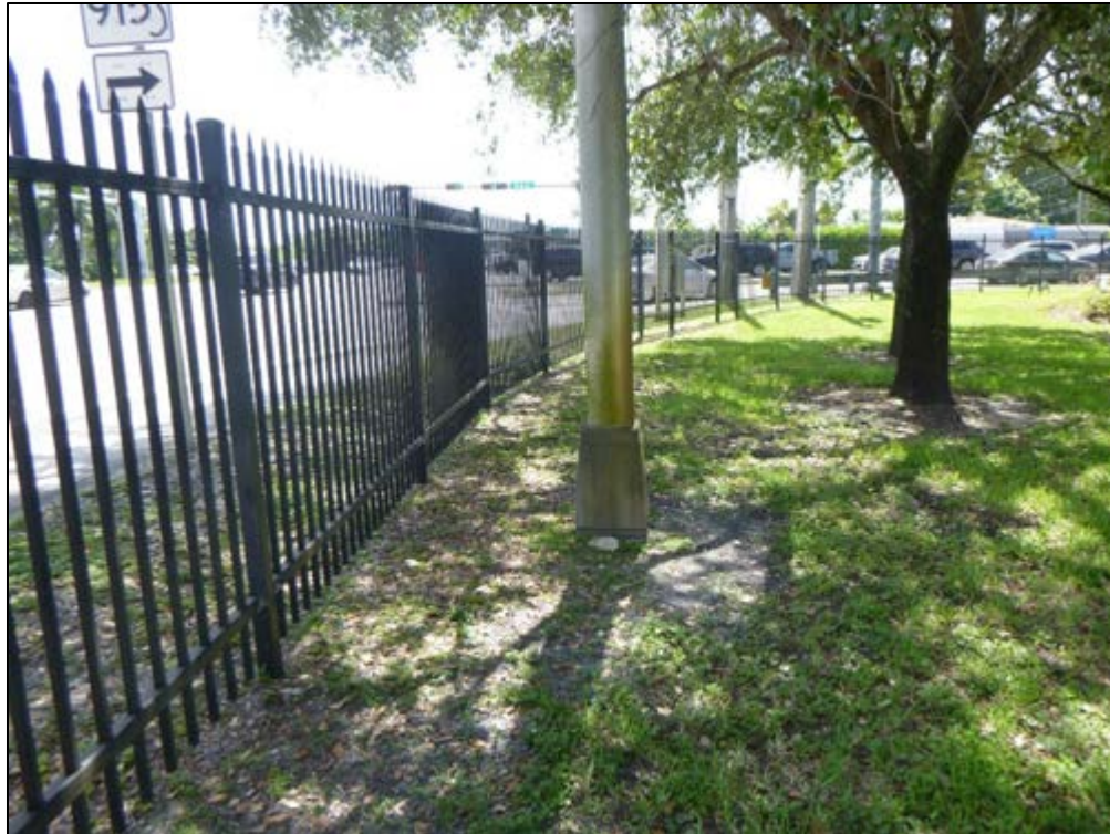
Figure 11 – 5: Buried Lighting Utilities and Fence within the Archaeological APE along Miami Gardens Drive East of I-95, Facing East
