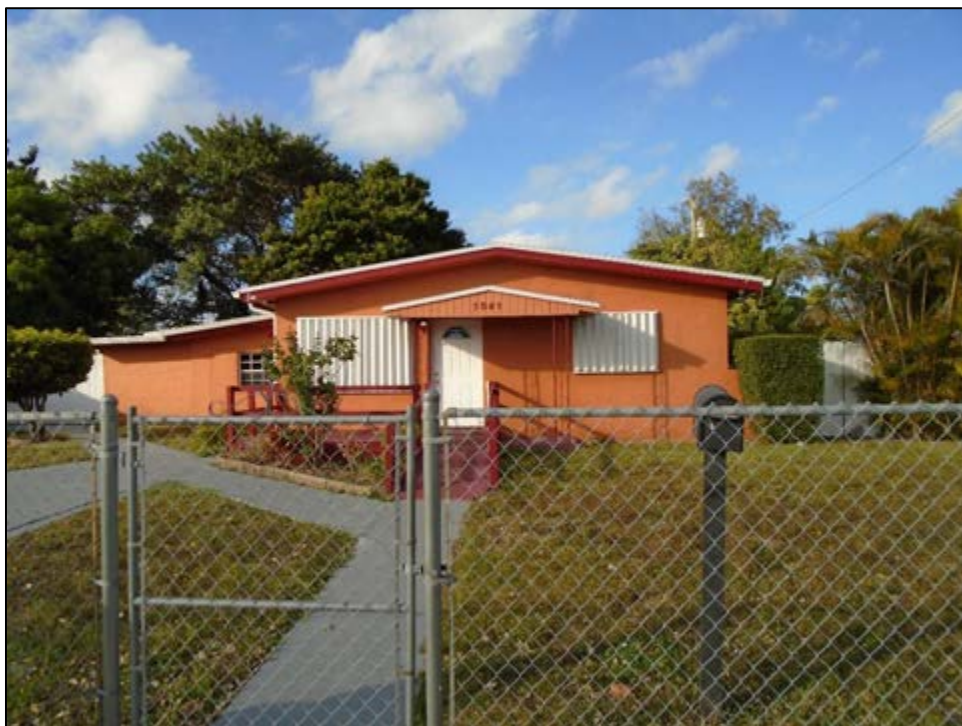
Figure 11 – 158: 1541 NE 205 th Terrace (8DA21465), c. 1956, Considered National Register-Ineligible, facing North
