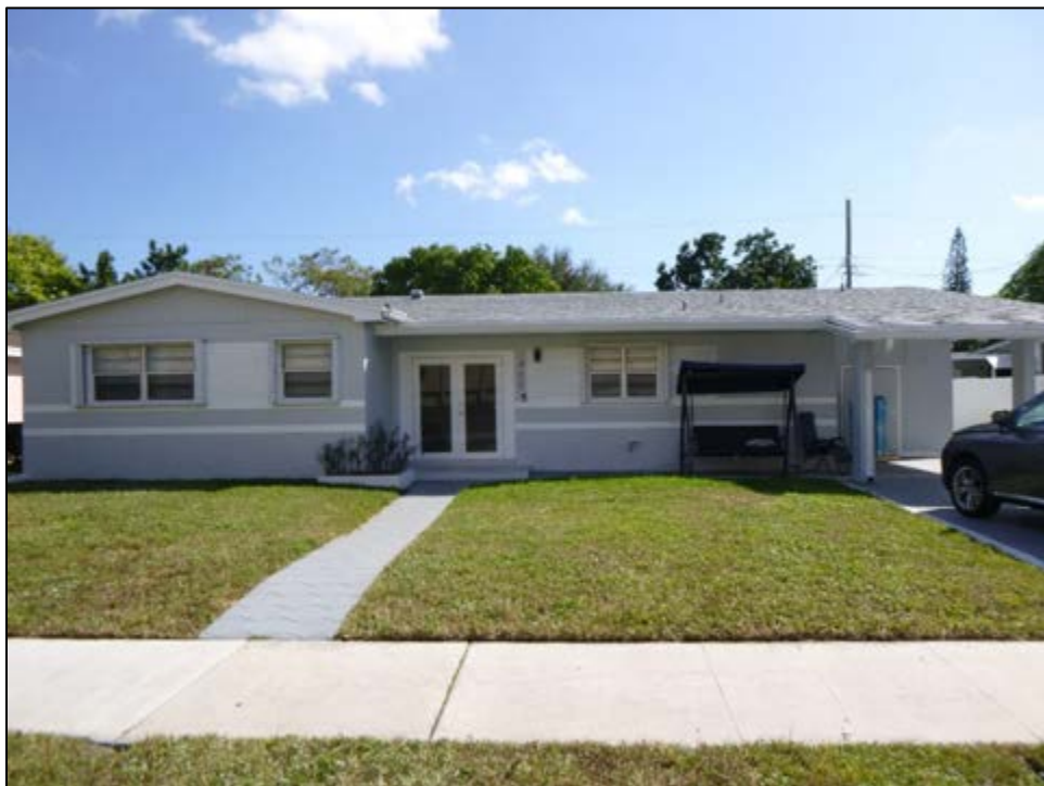
Figure 11 – 41: 420 East Drive (8DA14246), Determined National Register-Ineligible, facing Southeast
