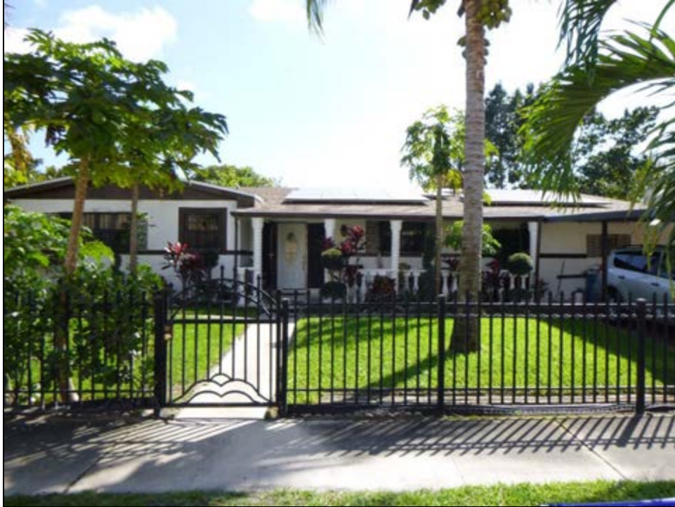
Figure 11 – 22: 200 East Drive (8DA14227), Determined National Register-Ineligible, facing Southeast
