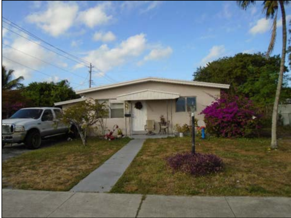
Figure 11 – 161: 1511 NE 205 th Terrace (8DA21468), c. 1956, Considered National Register-Ineligible, facing North
