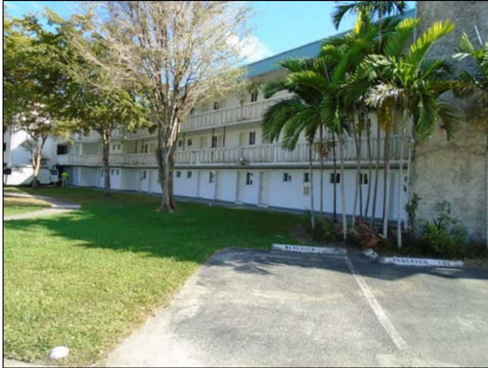
Figure 11 – 211: Riviera Condo Apartments (1170 NE 191 st Street) (8DA21540), c. 1966, Considered National Register-Ineligible, facing East
