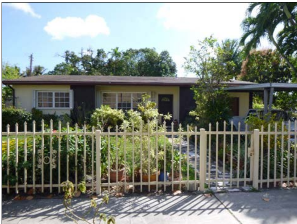
Figure 11 – 19: 170 East Drive (8DA14224), Determined National Register-Ineligible, facing Southeast
