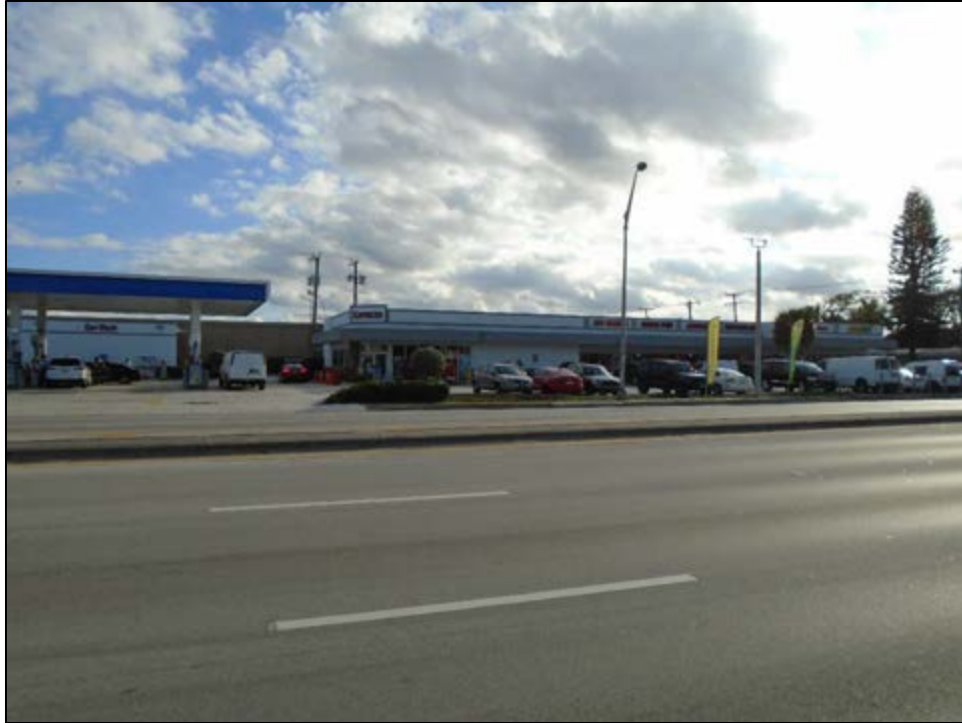
Figure 11 – 163: 1510 NE 205 th Street (8DA21470), c. 1959, Considered National Register-Ineligible, facing Southwest
