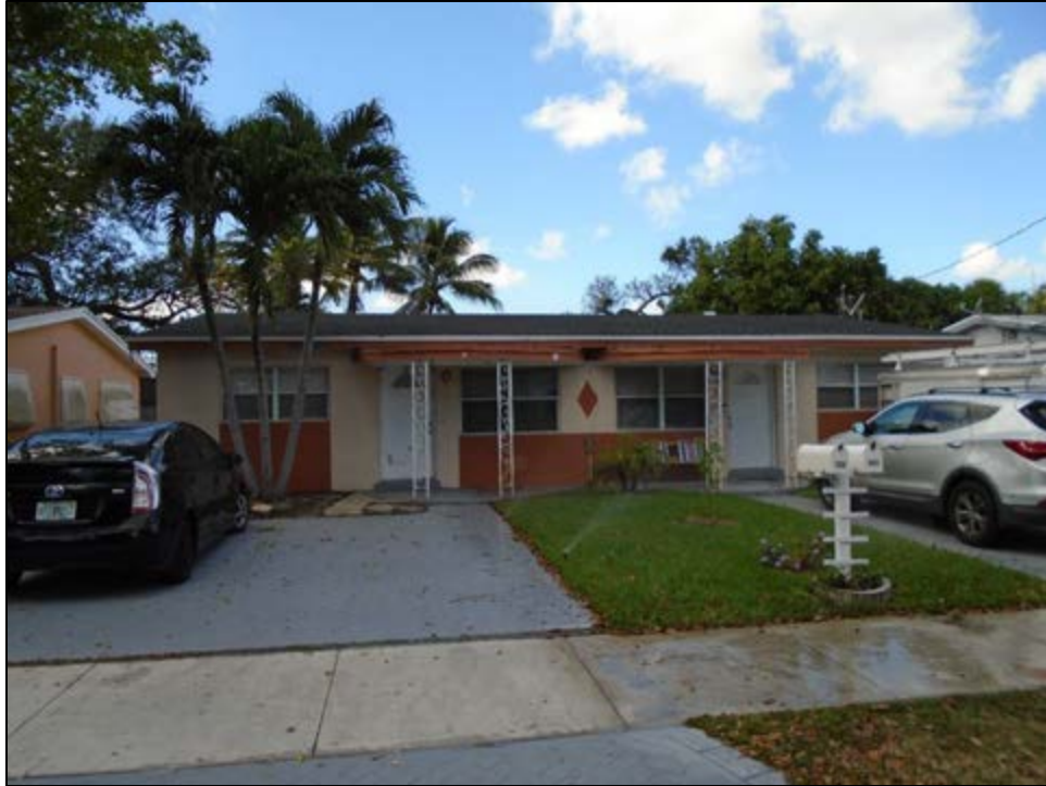
Figure 11 – 256: 310-312 SW 11 th Avenue (8BD8600), c. 1962, Considered National Register-Ineligible, facing West
