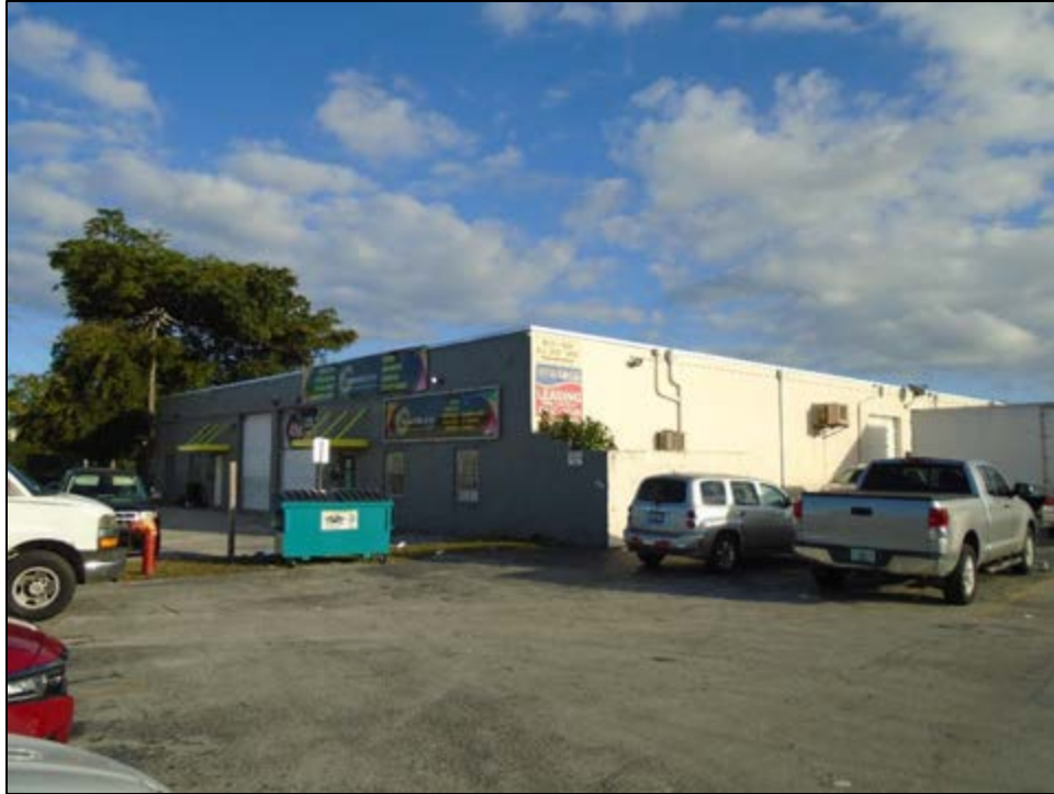
Figure 11 – 220: Ronson Industrial Park (1640 NE 205 th Terrace) (8DA21543), c. 1973, Considered National Register-Ineligible, facing Southeast
