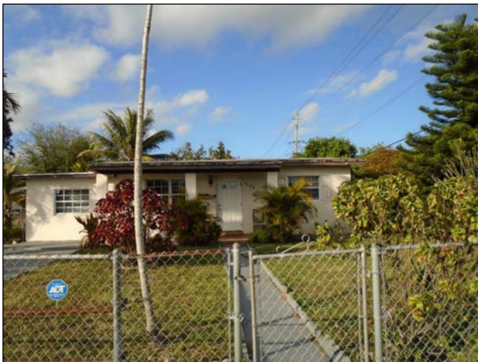
Figure 11 – 162: 1505 NE 205 th Terrace (8DA21469), c. 1955, Considered National Register-Ineligible, facing North
