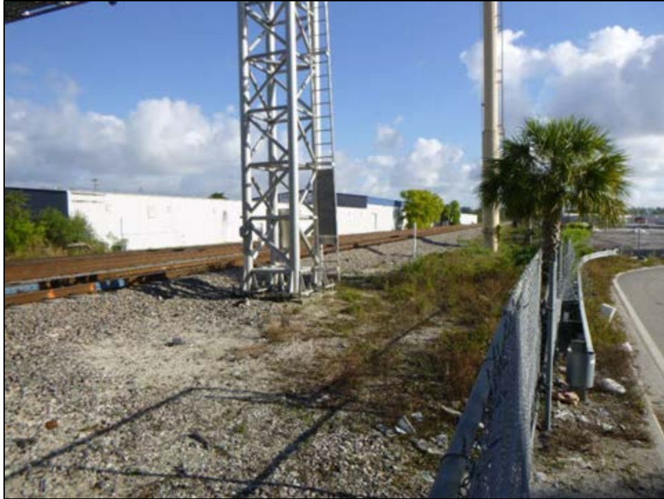
Figure 11 – 12: CSX Railroad (8DA10753) Within APE, Determined National Register-Eligible, facing Northeast
