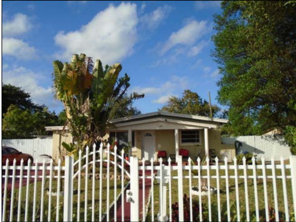
Figure 11 – 157: 1551 NE 205 th Terrace (8DA21464), c. 1956, Considered National Register-Ineligible, facing North
