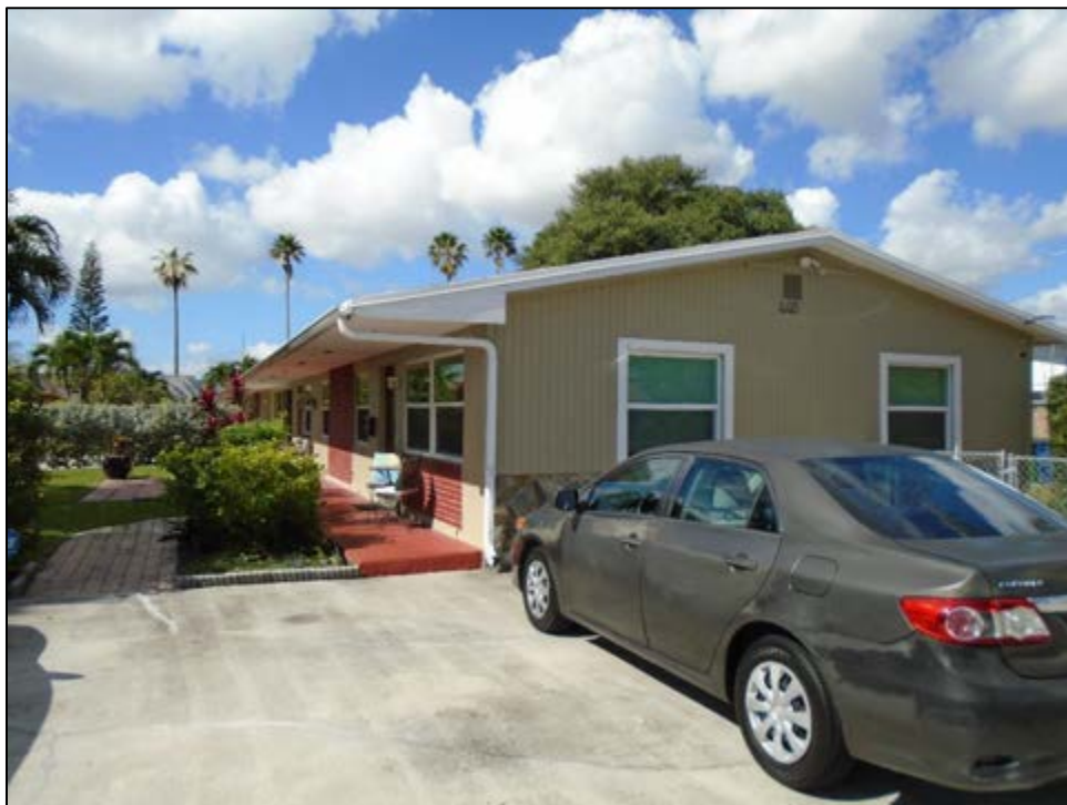
Figure 11 – 247: 440 SW 11 th Avenue (8BD8592), c. 1972, Considered National Register-Ineligible, facing West
