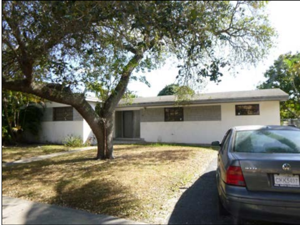
Figure 11 – 34: 340 East Drive (8DA14239), Determined National Register-Ineligible, facing Southeast
