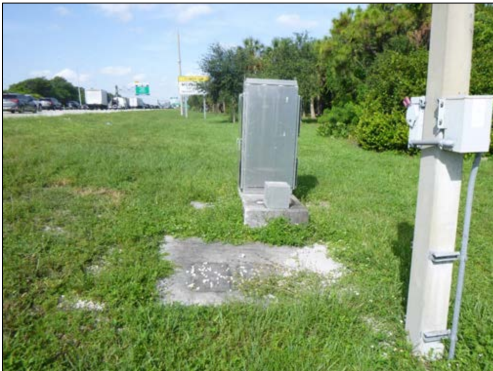
Figure 11 – 8: Buried Utilities and Exposed Road Fill in the Archaeological APE on the Western I-95 ROW across from the Moderate Probability Area, Facing Southwest
