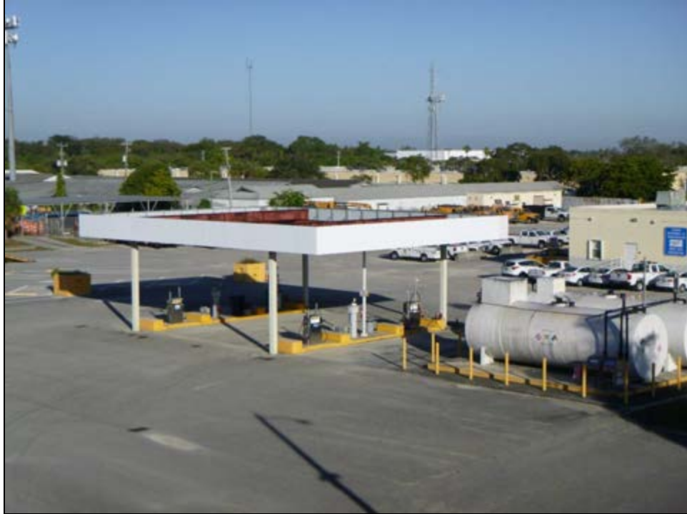
Figure 11 – 222: FDOT North Dade Maintenance Yard (1773 NE 205 th Street) (8DA21544), c. 1968, Considered National Register-Ineligible, facing Northwest
