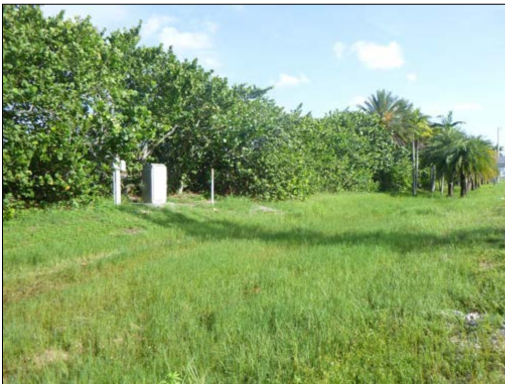
Figure 11 – 6: Berm, Ditch, Utilities, and Exposed Road Fill in the Archaeological APE on the Western I-95 ROW near the north end of the APE, Facing Northwest
