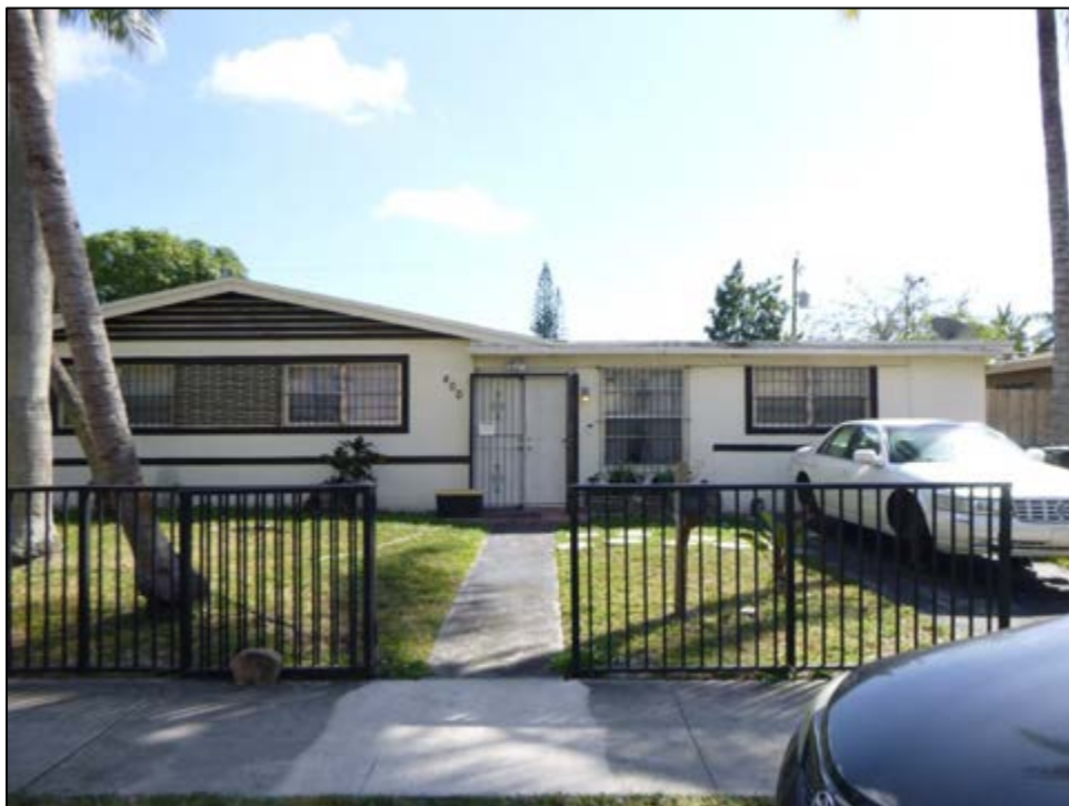
Figure 11 – 39: 400 East Drive (8DA14244), Determined National Register-Ineligible, facing Southeast
