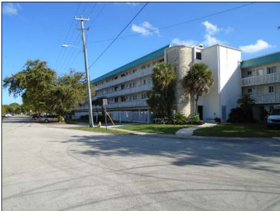
Figure 11 – 212: Riviera Condo Apartments (1170 NE 191 st Street) (8DA21540), c. 1966, Considered National Register-Ineligible, facing East
