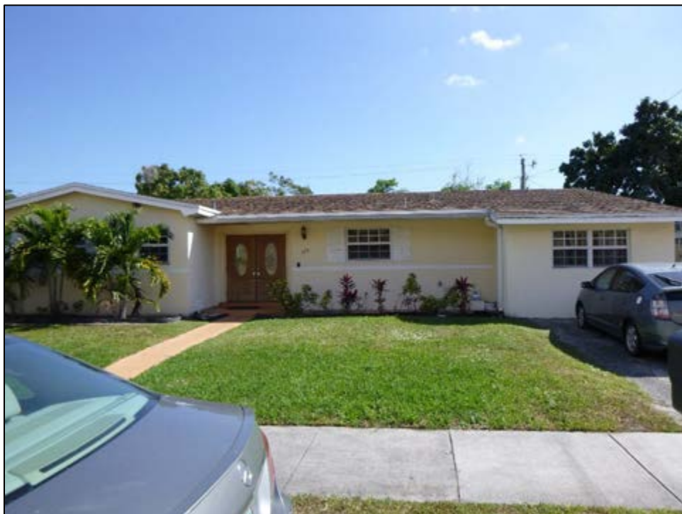
Figure 11 – 51: 520 East Drive (8DA14256), Determined National Register-Ineligible, facing Southeast
