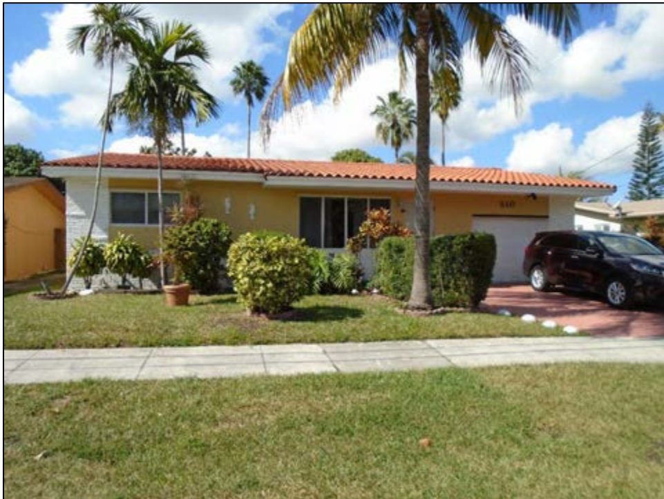
Figure 11 – 245: 510 SW 11 th Avenue (8BD8590), c. 1961, Considered National Register-Ineligible, facing West
