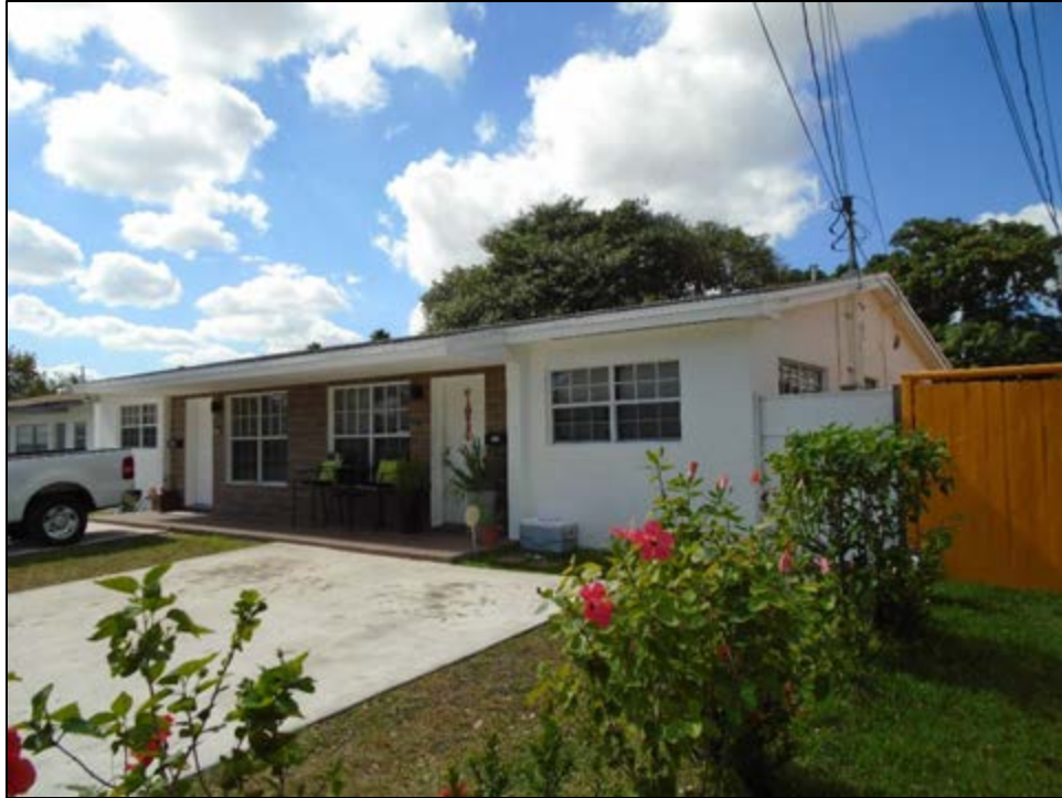
Figure 11 – 250: 420-422 SW 11 th Avenue (8BD8594), c. 1963, Considered National Register-Ineligible, facing Southwest
