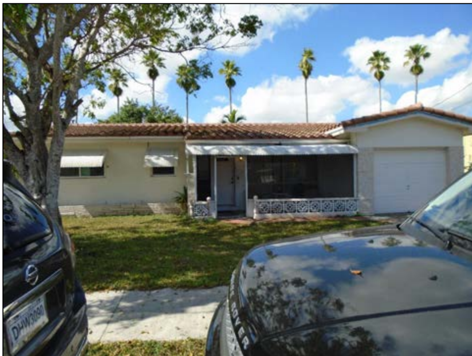
Figure 11 – 241: 600 SW 11 th Avenue (8BD8586), c. 1961, Considered National Register-Ineligible, facing West
