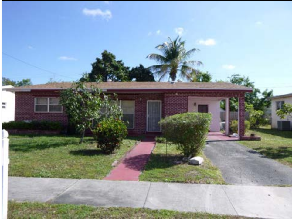
Figure 11 – 50: 510 East Drive (8DA14255), Determined National Register-Ineligible, facing Southeast
