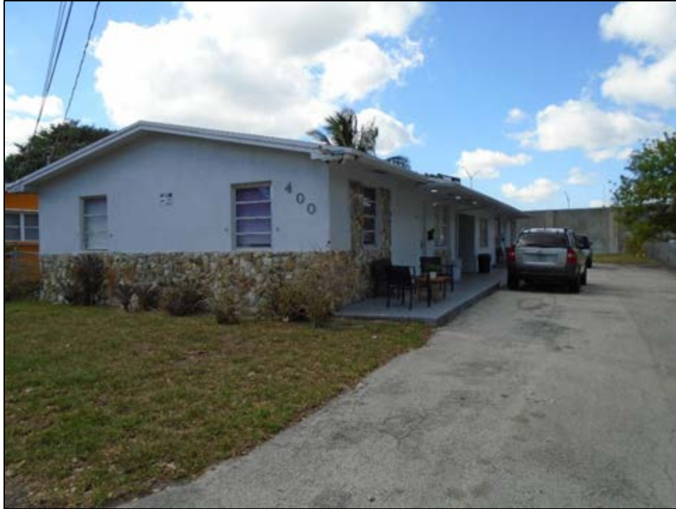
Figure 11 – 252: 400 SW 11 th Avenue (8BD8596), c. 1961, Considered National Register-Ineligible, facing Southwest
