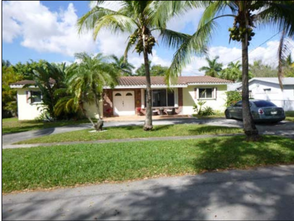
Figure 11 – 135: 18540 NE 7 th Court (8DA21445), c. 1964, Considered National Register-Ineligible, facing Northwest
