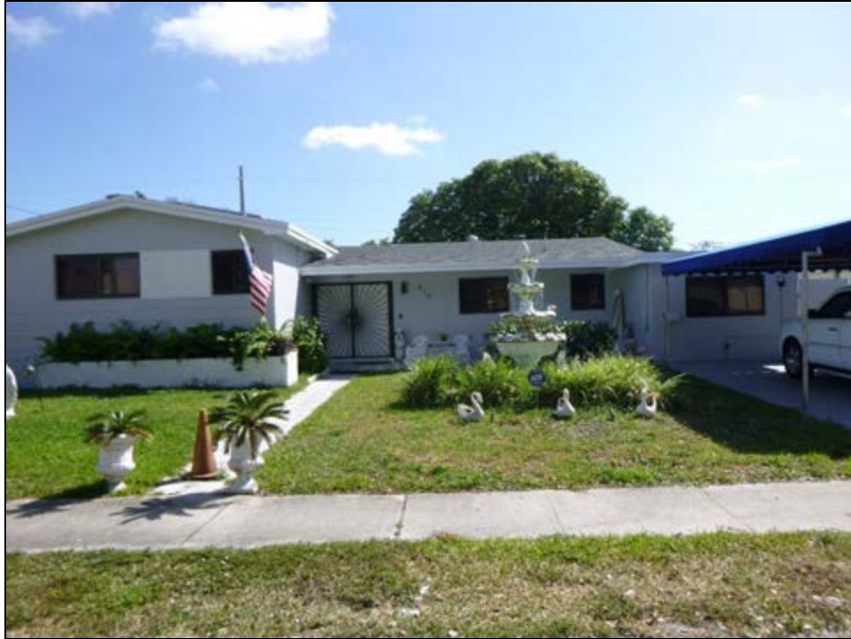
Figure 11 – 40: 410 East Drive (8DA14245), Determined National Register-Ineligible, facing Southeast
