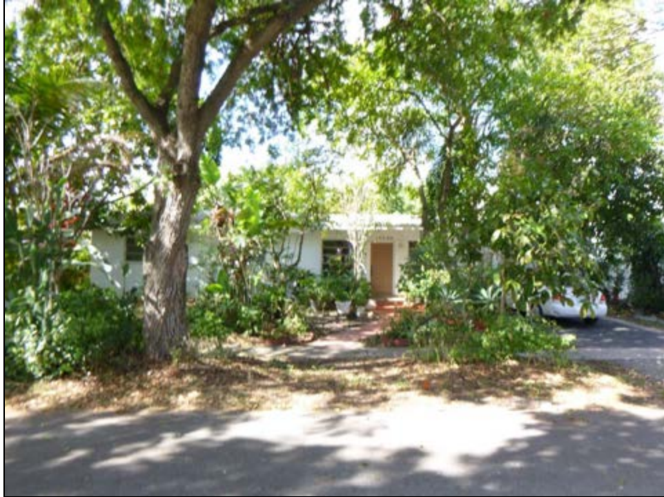
Figure 11 – 60: 18320 NE 7 th Court (8DA14269), Determined National Register-Ineligible, facing West
