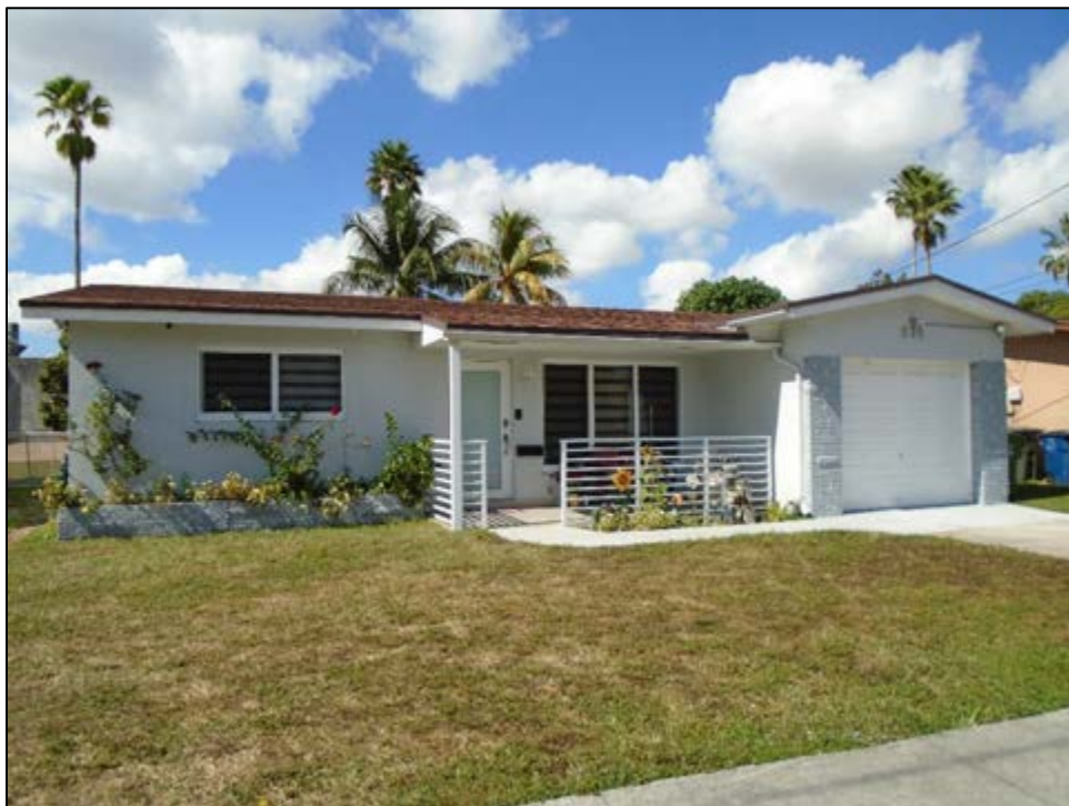
Figure 11 – 243: 530 SW 11 th Avenue (8BD8588), c. 1962, Considered National Register-Ineligible, facing West
