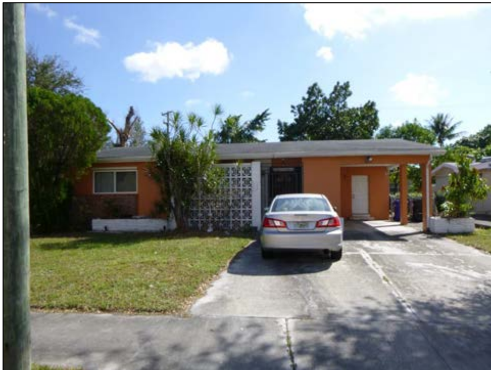
Figure 11 – 21: 190 East Drive (8DA14226), Determined National Register-Ineligible, facing Southeast
