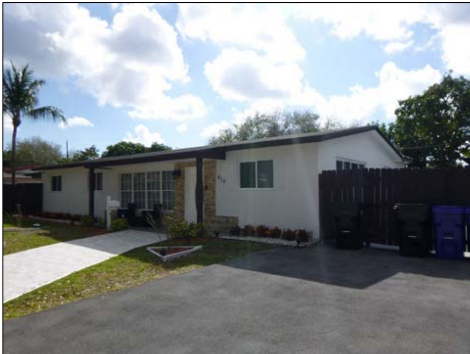
Figure 11 – 124: 810 NE 182 nd Street (8DA21434), c. 1964, Considered National Register-Ineligible, facing Southeast
