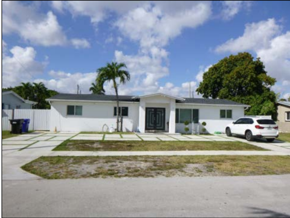
Figure 11 – 62: 18360 NE 7 th Court (8DA14271), Determined National Register-Ineligible, facing West
