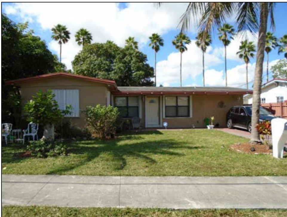
Figure 11 – 237: 640 SW 11 th Avenue (8BD8582), c. 1961, Considered National Register-Ineligible, facing West
