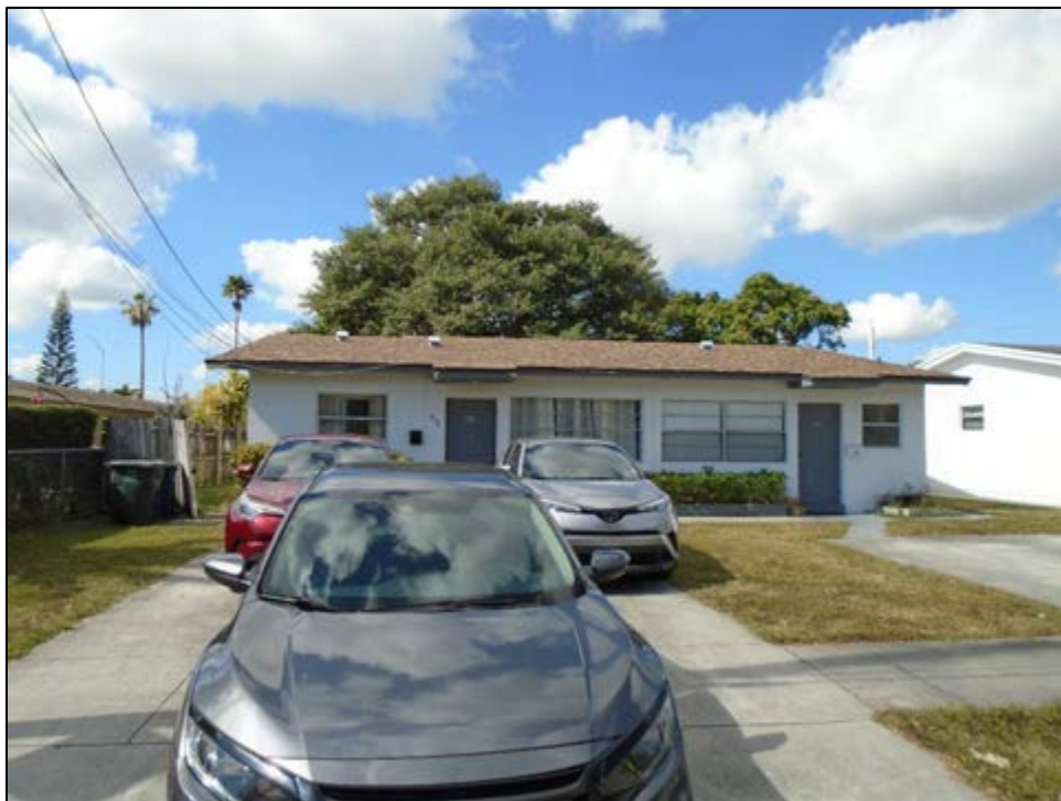
Figure 11 – 249: 430-434 SW 11 th Avenue (8BD8593), c. 1963, Considered National Register-Ineligible, facing West
