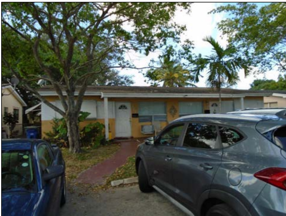
Figure 11 – 255: 320-322 SW 11 th Avenue (8BD8599), c. 1962, Considered National Register-Ineligible, facing West
