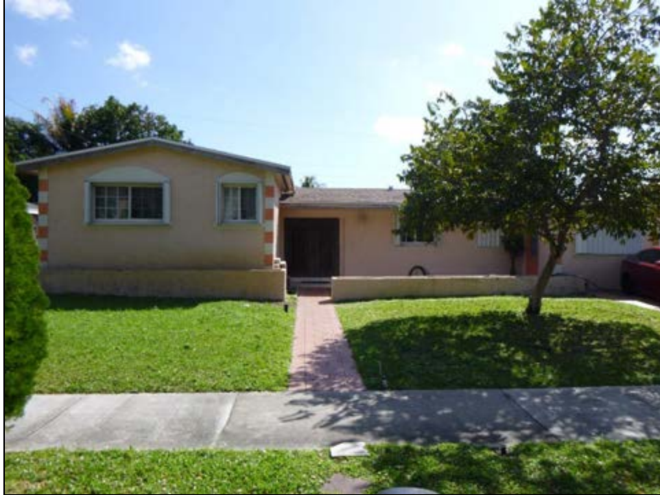
Figure 11 – 32: 320 East Drive (8DA14237), Determined National Register-Ineligible, facing Southeast
