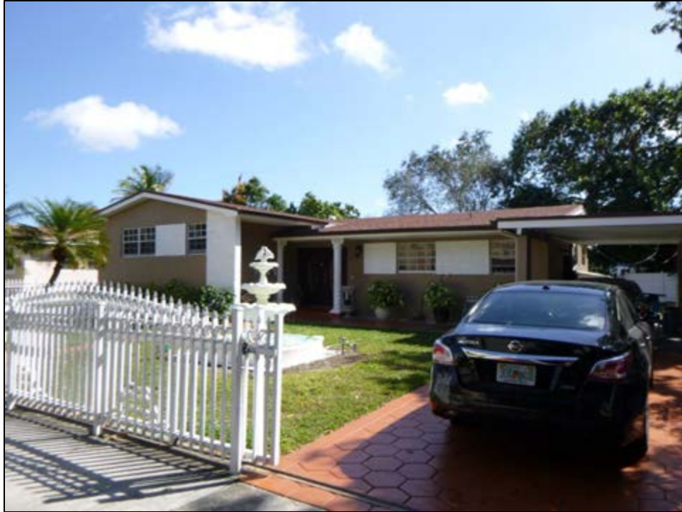
Figure 11 – 28: 270 East Drive (8DA14233), Determined National Register-Ineligible, facing Southeast
