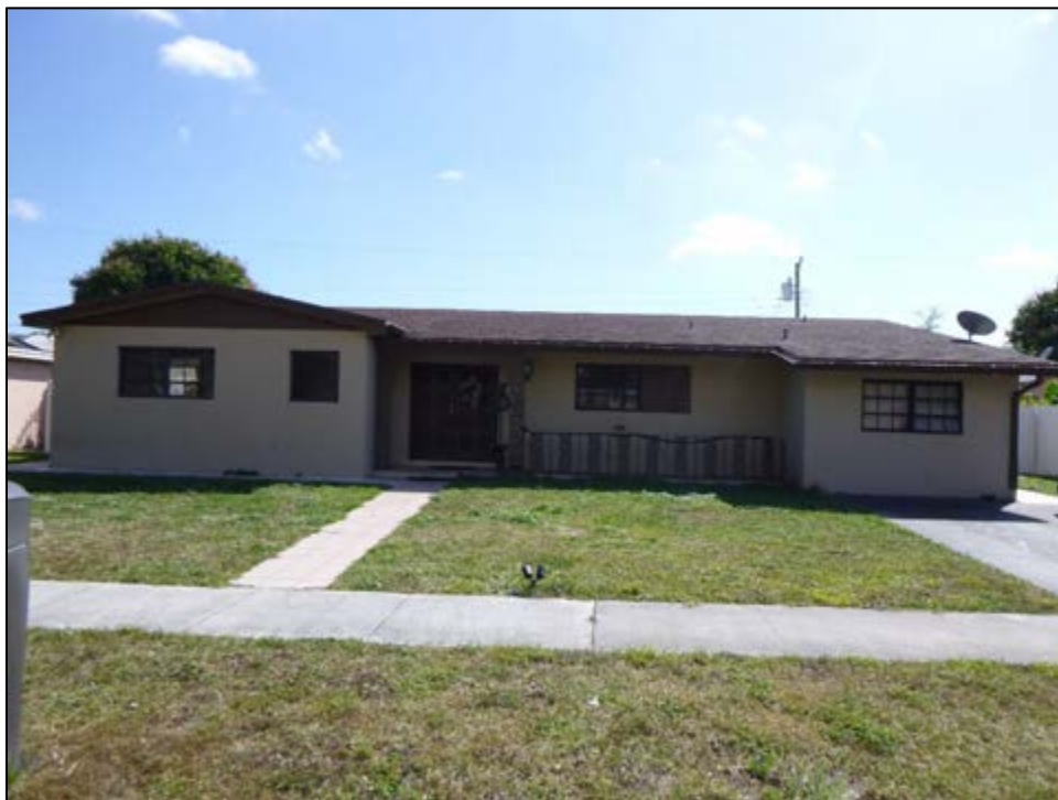
Figure 11 – 31: 310 East Drive (8DA14236), Determined National Register-Ineligible, facing Southeast
