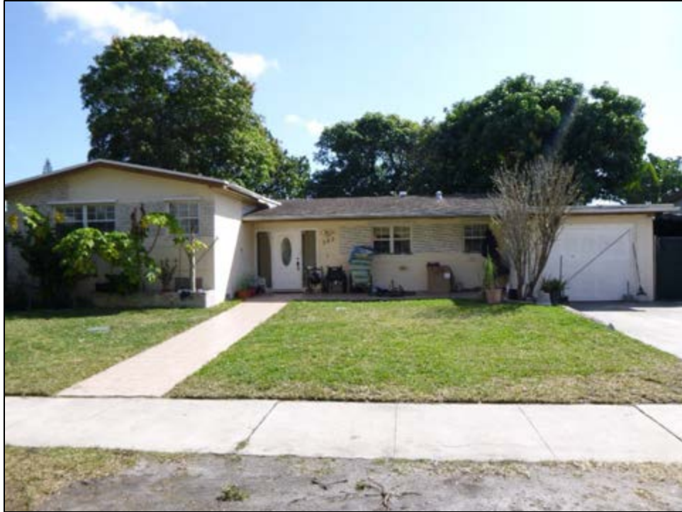
Figure 11 – 36: 360 East Drive (8DA14241), Determined National Register-Ineligible, facing Southeast
