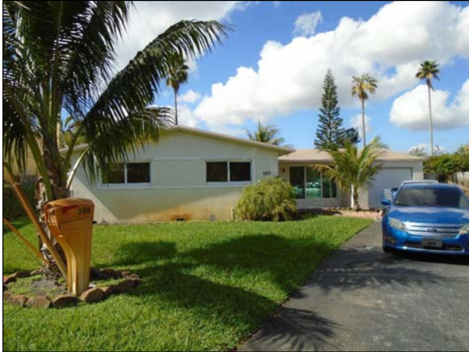
Figure 11 – 246: 500 SW 11 th Avenue (8BD891), c. 1960, Considered National Register-Ineligible, facing West
