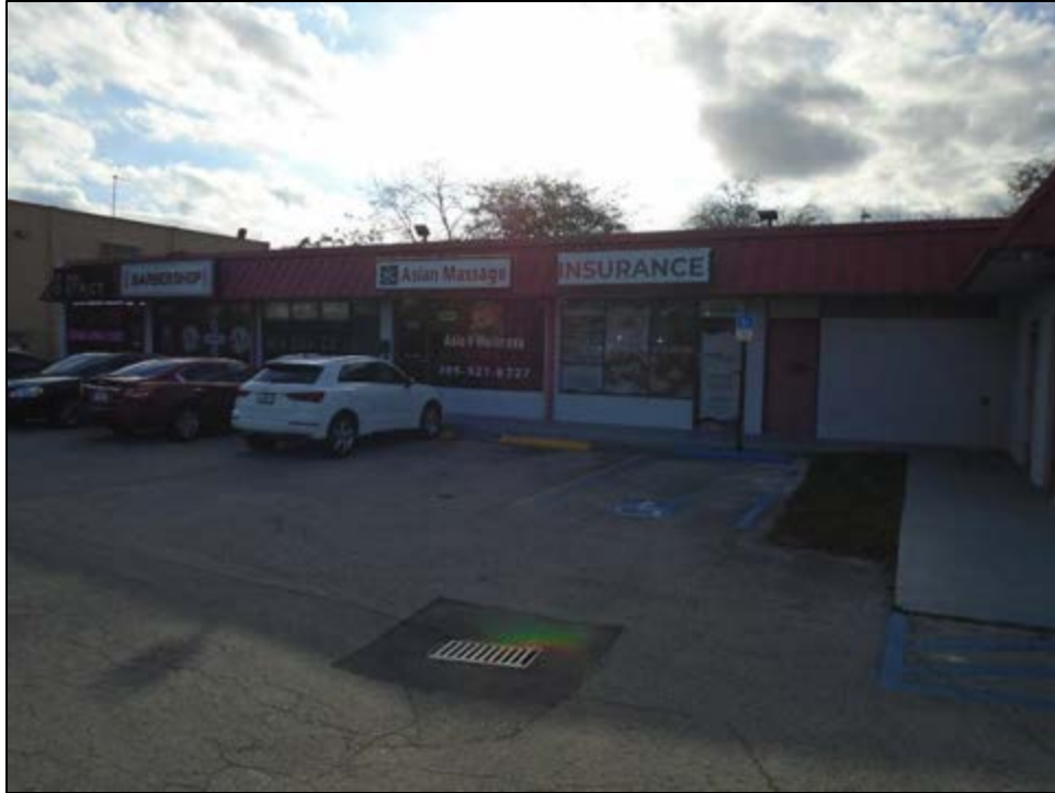
Figure 11 – 165: 1560 NE 205 th Street (8DA21471), c. 1974, Considered National Register-Ineligible, facing Southwest
