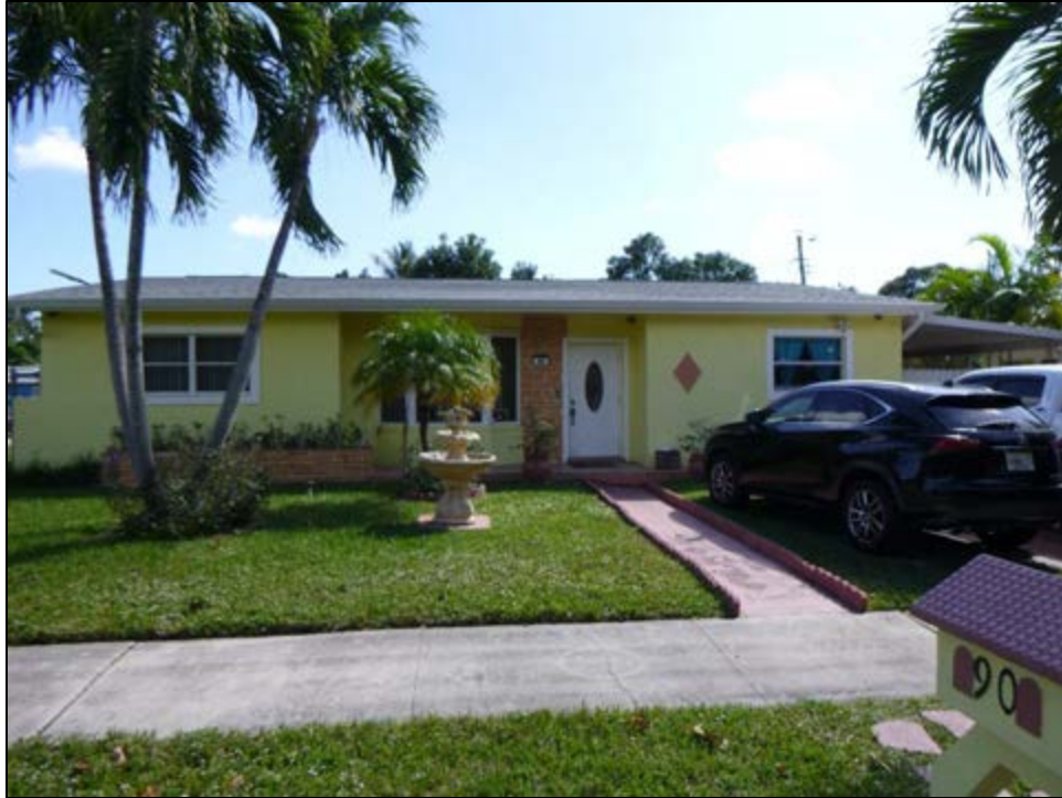
Figure 11 – 66: 90 East Drive (8DA14278), Determined National Register-Ineligible, facing Southeast
