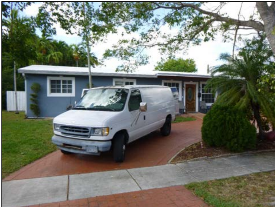
Figure 11 – 130: 18200 NE 7 th Court (8DA21440), c. 1963, Considered National Register-Ineligible, facing Northwest
