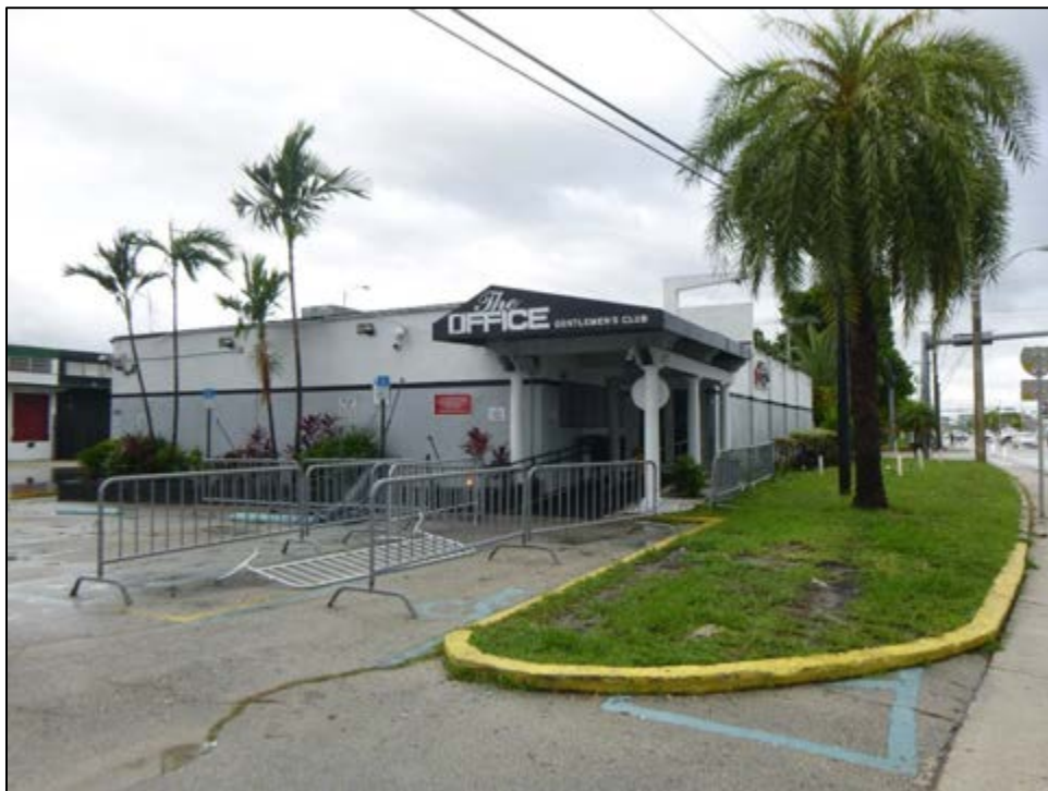
Figure 11 – 112: 290 NE 183 rd Street (8DA21423) Outparcel Building, c. 1966, Considered National Register-Ineligible, facing Southwest
