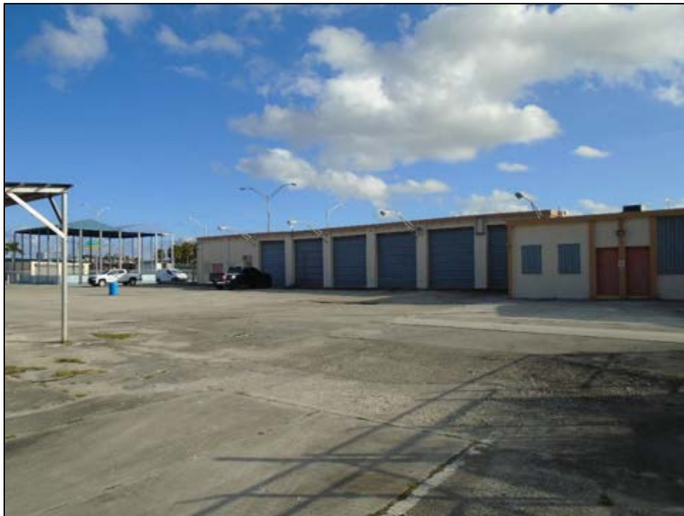
Figure 11 – 154: Miami Dade Fire Rescue Station #63 (1655 NE 205 th Street) (8DA21461), c. 1968, Considered National Register-Ineligible, facing Southeast
