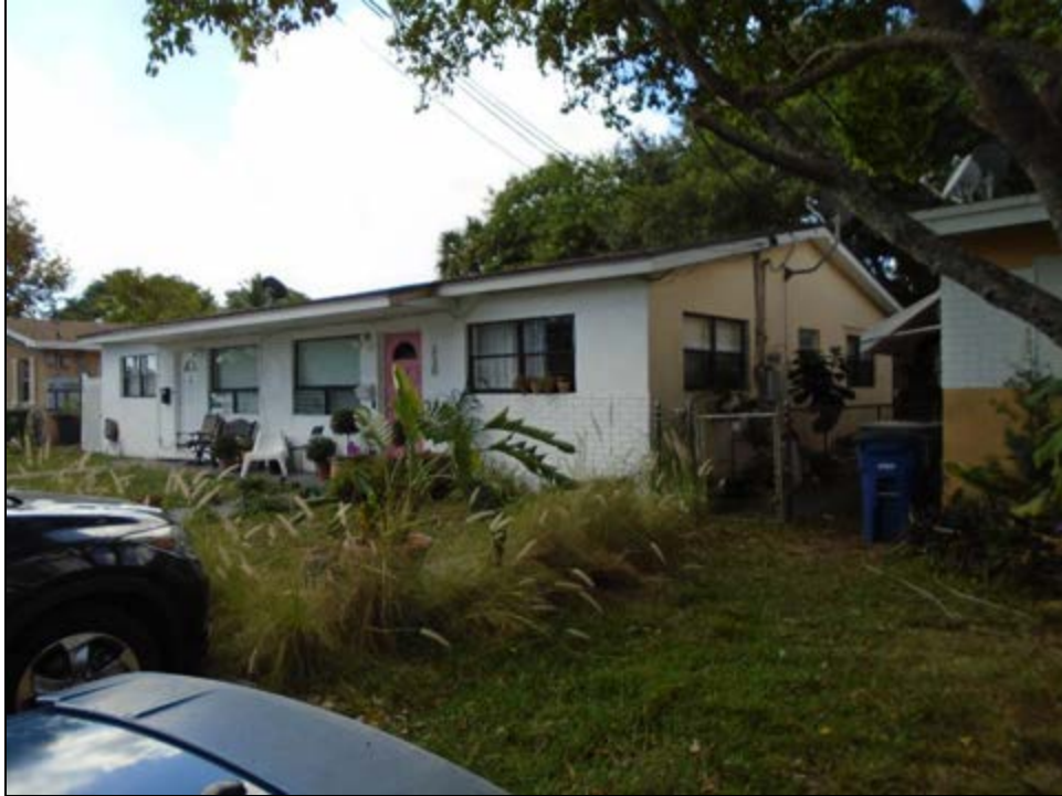
Figure 11 – 254: 330-332 SW 11 th Avenue (8BD8598), c. 1962, Considered National Register-Ineligible, facing Southwest
