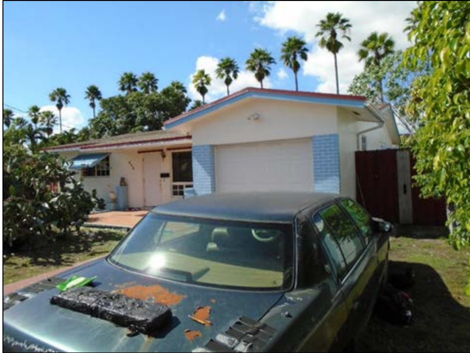
Figure 11 – 238: 630 SW 11 th Avenue (8BD8583), c. 1962, Considered National Register-Ineligible, facing Southwest
