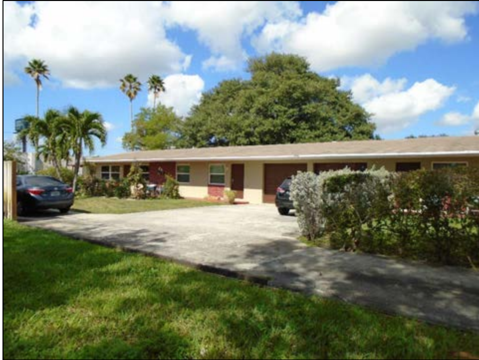
Figure 11 – 248: 440 SW 11 th Avenue (8BD8592), c. 1972, Considered National Register-Ineligible, facing Northwest
