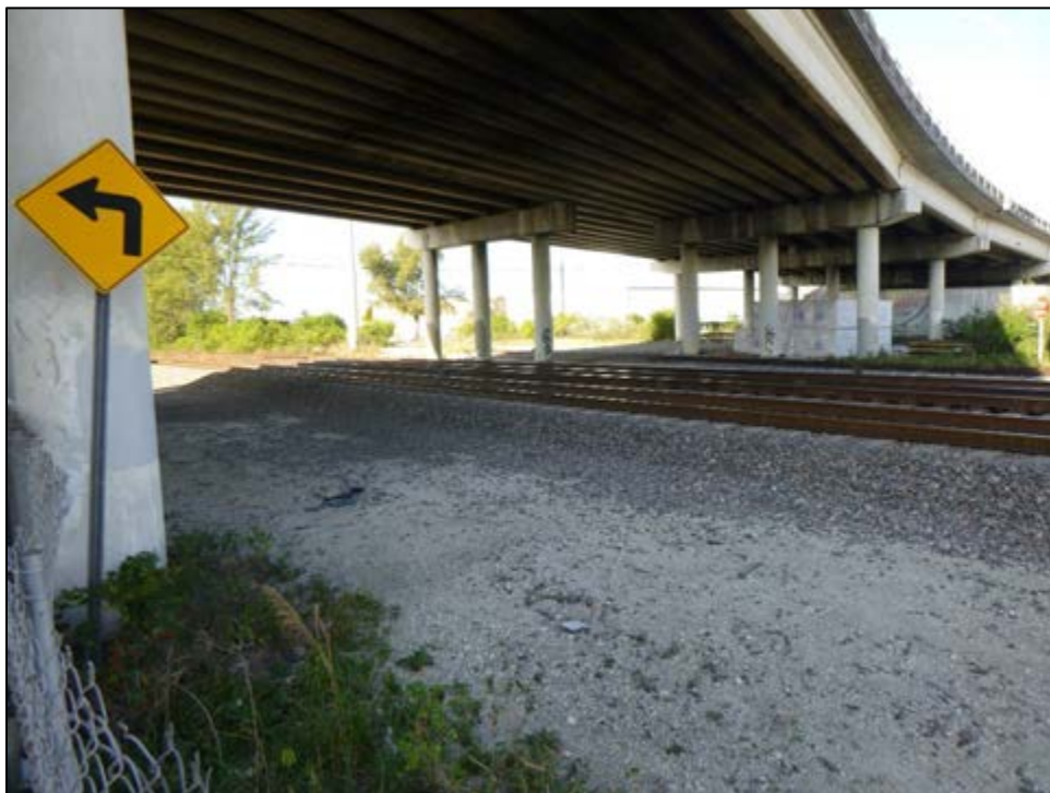
Figure 11 – 13: CSX Railroad (8DA10753) Within APE, Determined National Register-Eligible, facing Southwest
