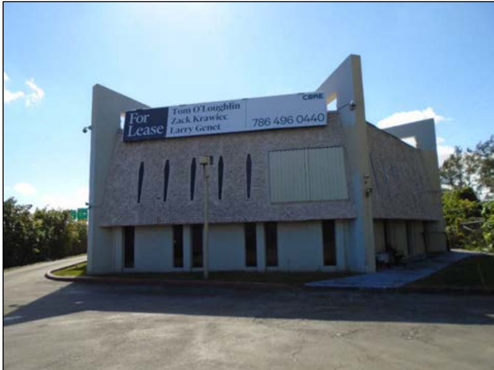
Figure 11 – 148: 18500 NE 5 th Avenue (8DA21460), c. 1971, Considered National Register-Ineligible, facing Southwest
