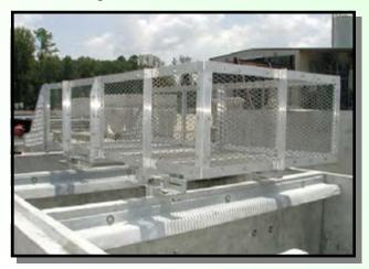
Turbulence deflectors are attached to the tops of the baffles with stainless steel bolts. Several bolts per deflector are required.
