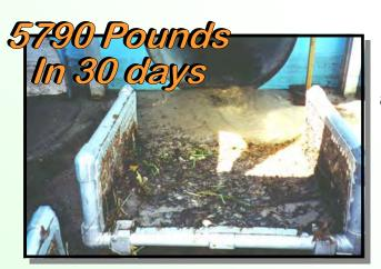
To the left is a view of 5790 pounds of sediment collected in a Nutrient Separating Baffle Box just 30 days after installation.
