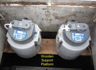
Figure 3-3. Overview of Sampling Equipment Installed at the Gee Creek Site.
