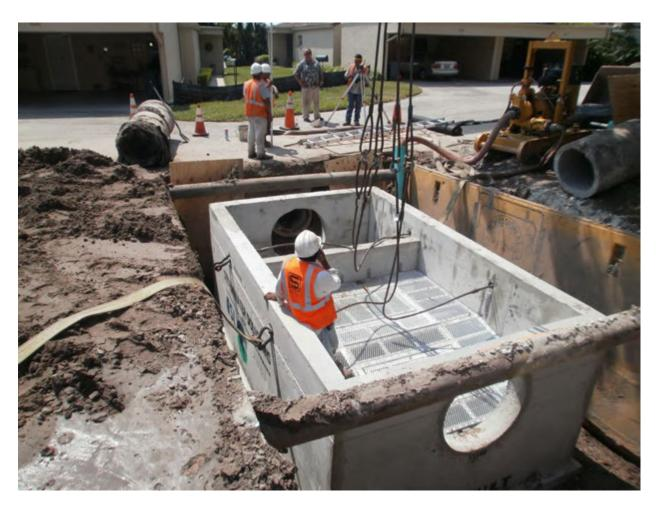
Installation of one of the smaller baffle boxes at the Sausalito Condos on Lake Howell. This box treats a 24" storm pipe – the upstream side is in the foreground (Lake Howell is just beyond the buildings in the photo.) The leaf screen can be seen on the upstream side of the box.
