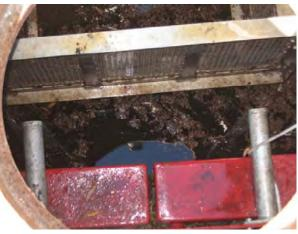
d. Baffle box unit following cleaning
