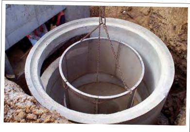
CDS removes fine sediments and trash debris
