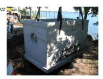
EcoVault® treats the continuous flow while debris screens span the entire box, creating extensive storage volume.
