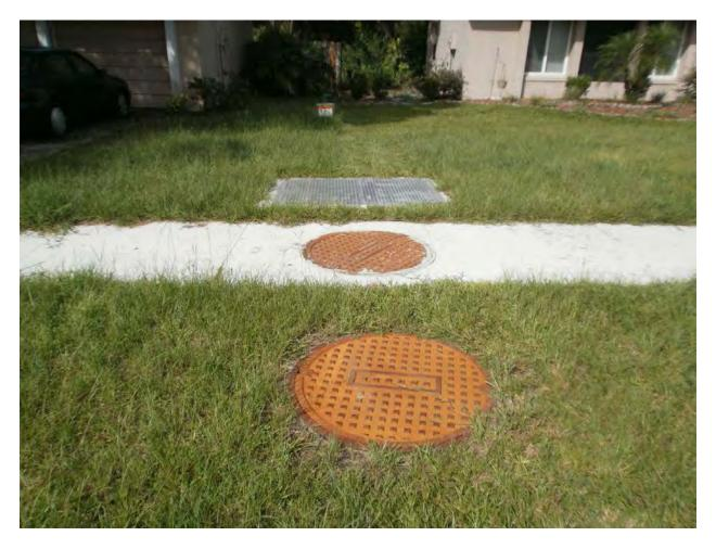
Baffle box on Osceola Trail at Gee Creek after full restoration. Gee Creek is behind the homes in the background. The manholes and hatches are used to access the baffle box for maintenance, including cleanouts and filter replacement.
