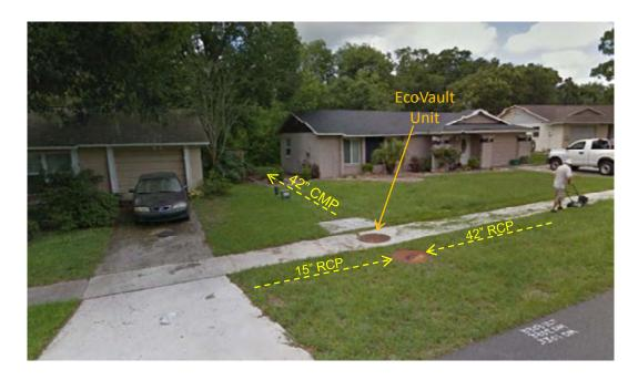
Figure 2-12. Photograph of the Exterior of the Gee Creek EcoVault® Unit.
