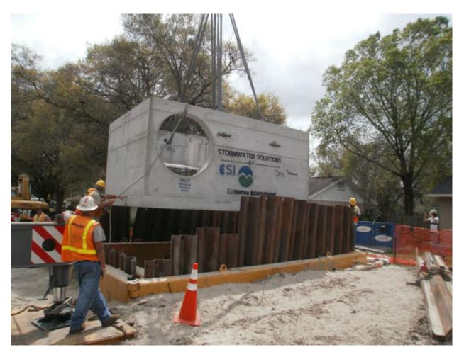
Lowering of one of the larger baffle boxes via crane on Osceola Trail at Gee Creek. Note the temporary sheet pile installation around the excavated area. The large opening in the side of the box is where the 42" upstream pipe was set (see next photo). Gee Creek (receiving water) is behind the homes to the right in the photo.
