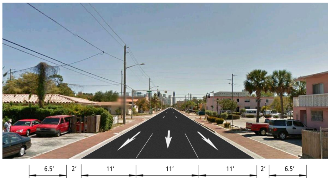
Figure 1-3: Existing Roadway Typical Section of Eastbound SR 90
