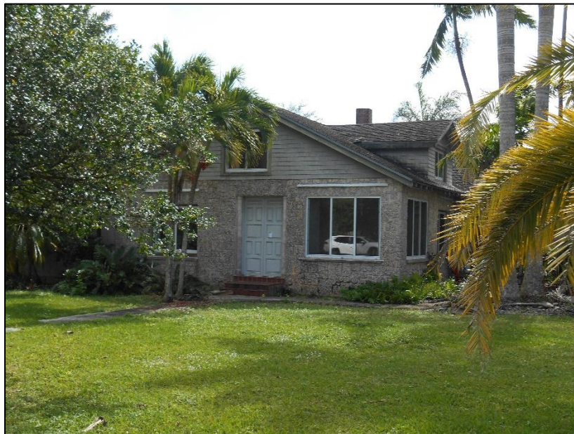
Figure 3-5: Northern elevation of the main house of the National Register–eligible and locally designated Talbott Estate (8DA2789). The doorway features thin oolitic limestone columns flanking the entrance, facing south
