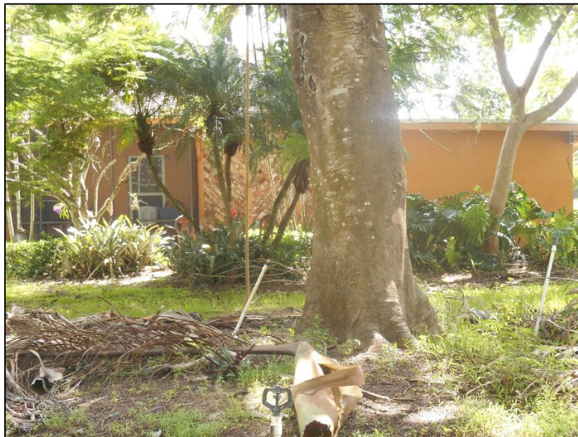
Figure 3-9: Western elevation of the cottage outbuilding south of the converted shed on the National Register–eligible and locally designated Talbott Estate (8DA2789). The decorative brickwork on the western wall of this building is visible in this photograph, facing east
