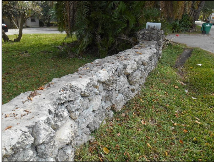
Figure 3-4: Oolitic limestone exterior wall, located at the western driveway entrance to the National Register–eligible and locally designated Talbott Estate (8DA2789). At this entrance, multiple mailboxes are incorporated into the wall, facing south
