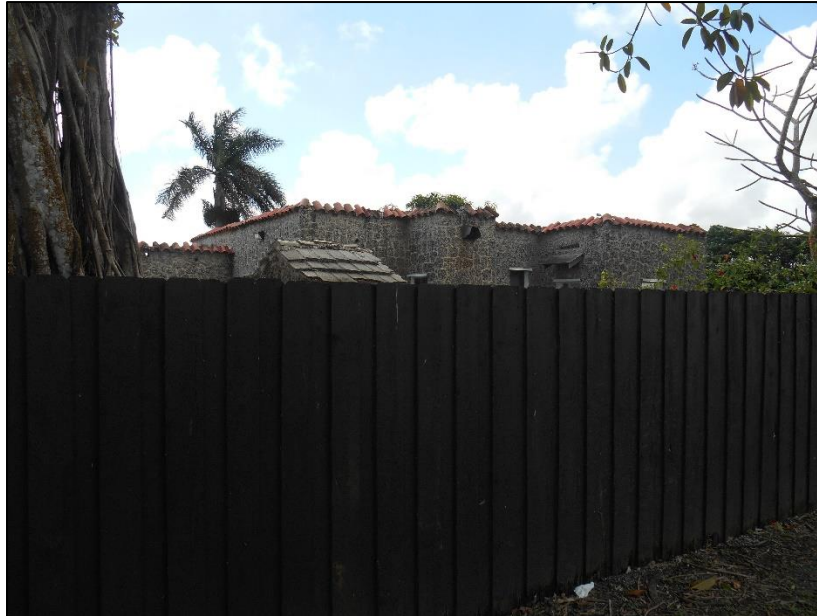
Figure 3-15: Northern elevation of the National Register–eligible building at 20000 SW 137th Avenue (8DA20713). The gabled topper of the parcel’s oolitic limestone wall is visible in the foreground, behind the privacy fence, facing south
