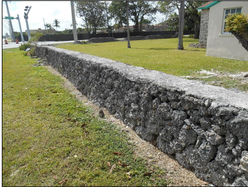
Figure 3-14: Segment of oolitic limestone exterior wall, located along eastern edge of the National Register–eligible MacDonell Residence (8DA20712, facing south)
