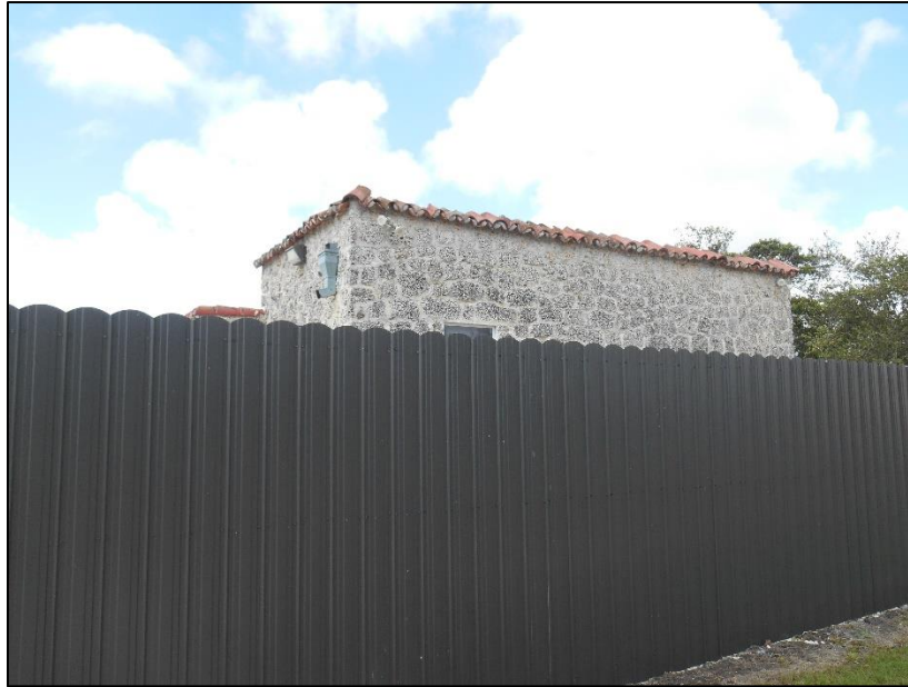
Figure 3-17: Eastern elevation of the southeastern outbuilding on the property containing the National Register–eligible building at 20000 SW 137th Avenue (8DA20713), facing west
