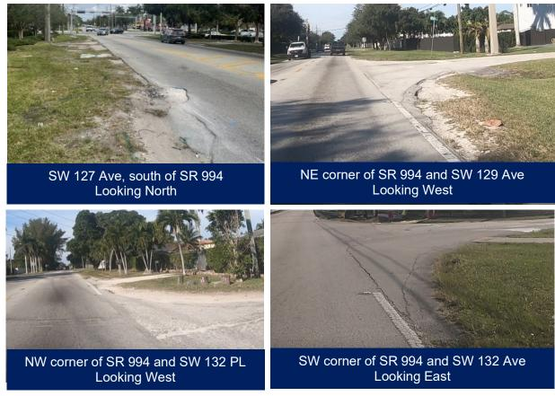
Figure 2-8 Existing Pavement Deficiencies
