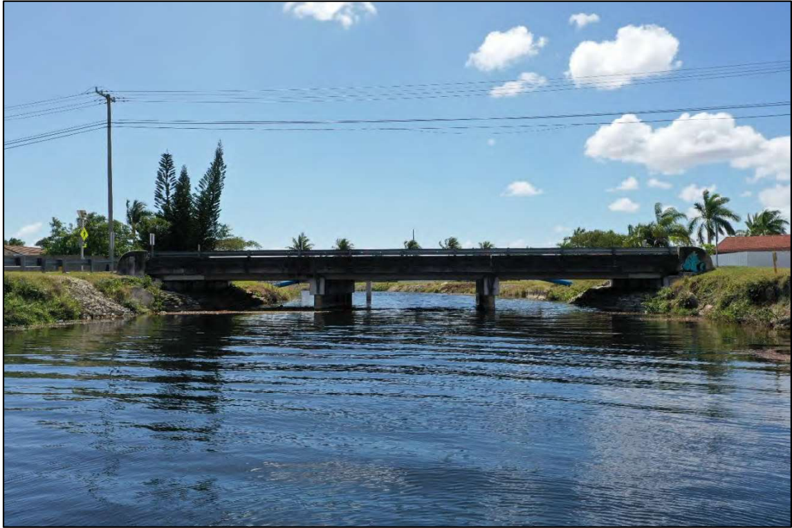
Photograph of Bridge Facing South
