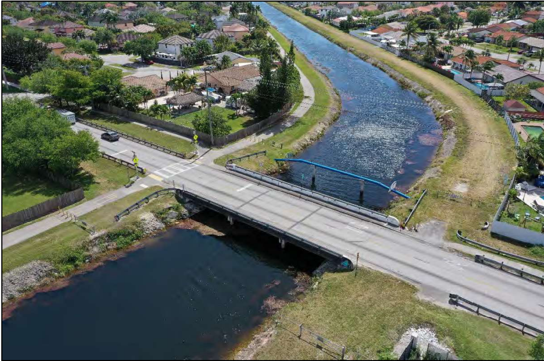
Aerial Photograph of the Black Creek Canal
