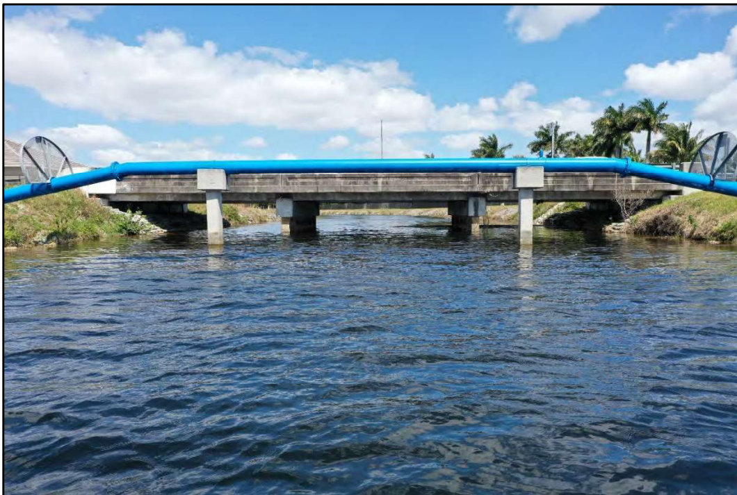
Photograph of Bridge Facing North
