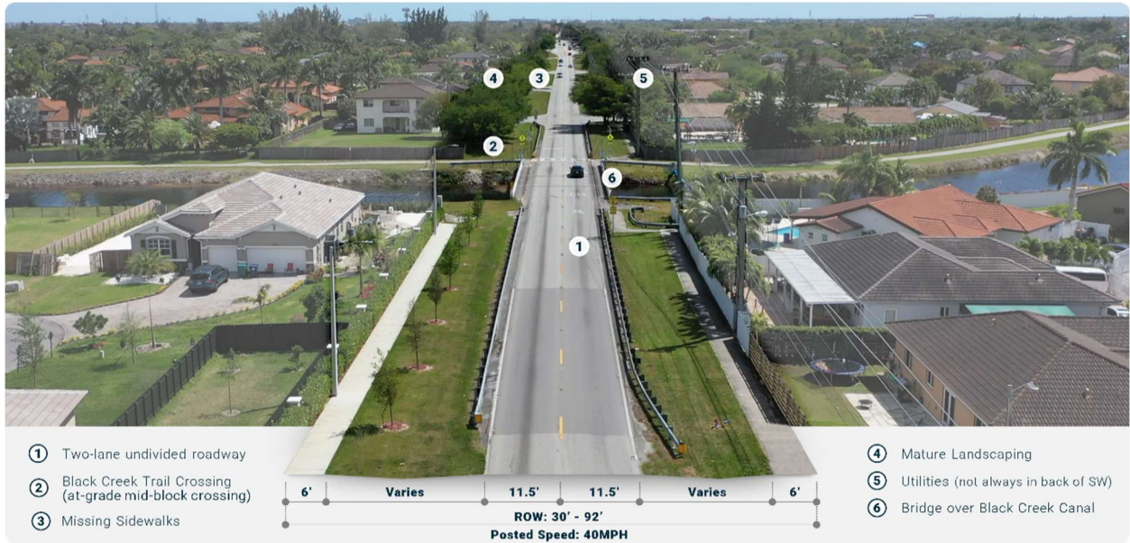
Figure 3-1: Existing Typical Section
