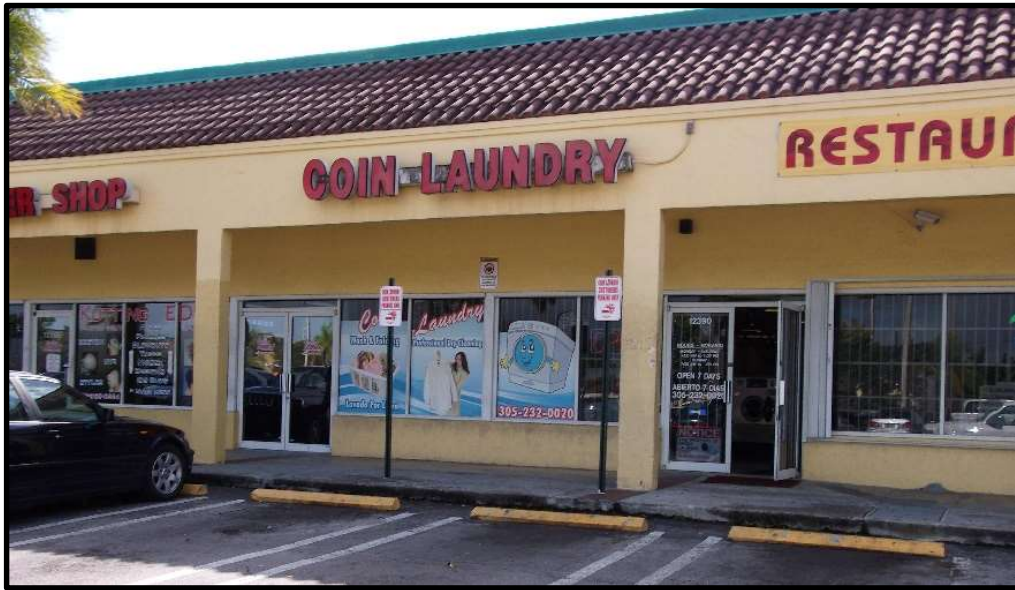
Photo 1: Contaminated Site - Coin Laundry
