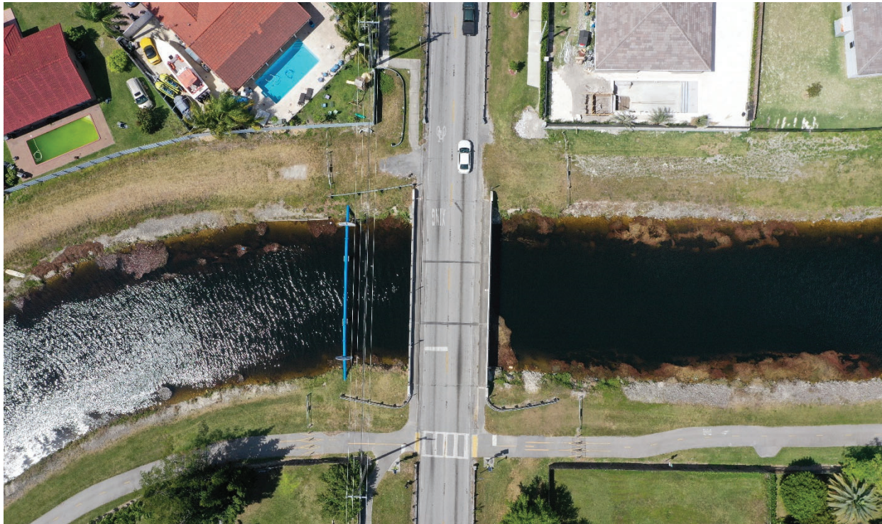
Figure 3 – Existing Bridge Aerial
