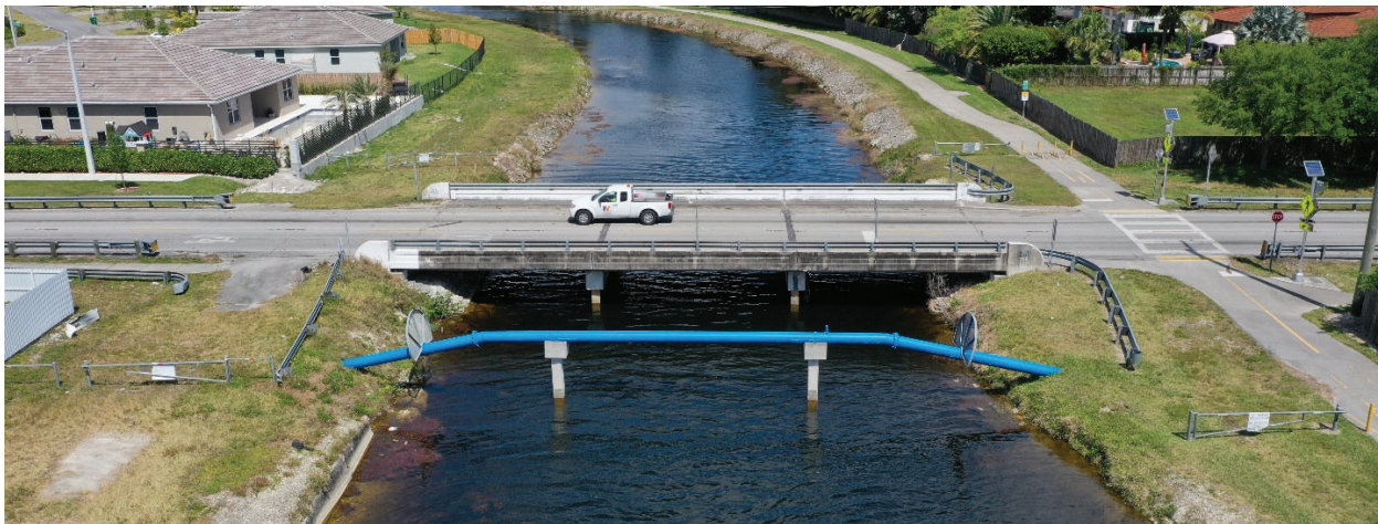
Figure 2 – Existing Bridge Elevation Looking North
